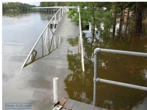
Figure 4-9. Boat Ramp and Courtesy Dock
