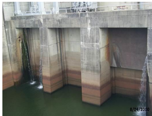
Figure 2-7. Draft Tube Gates
