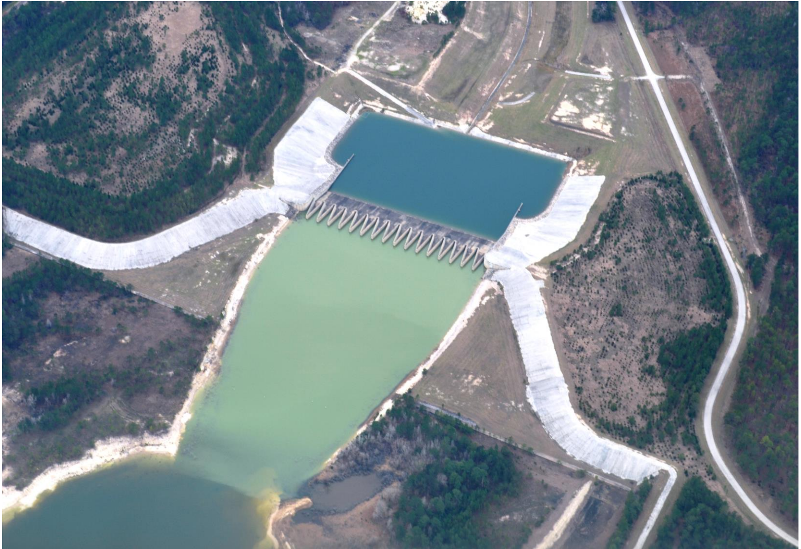
SAM RAYBURN DAM AND RESERVOIR
