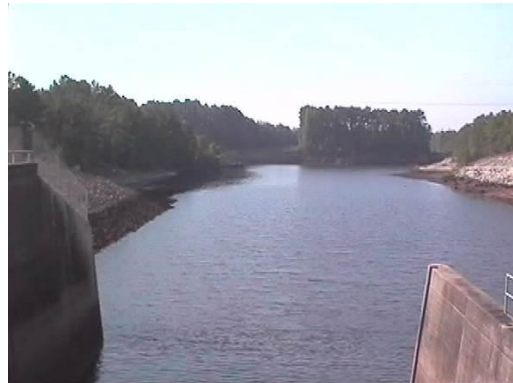
Figure 2-5. Outlet Works Stilling Basin and Discharge Channel
