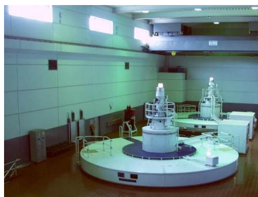
Figure 2-9. Powerhouse Generators
