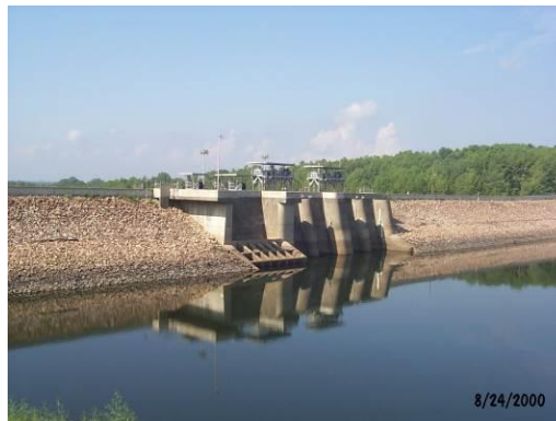
Figure 2-2. Upstream View of Embankment and Intake Structures
