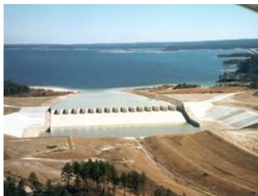
Figure 2-3. Aerial View of Spillway
