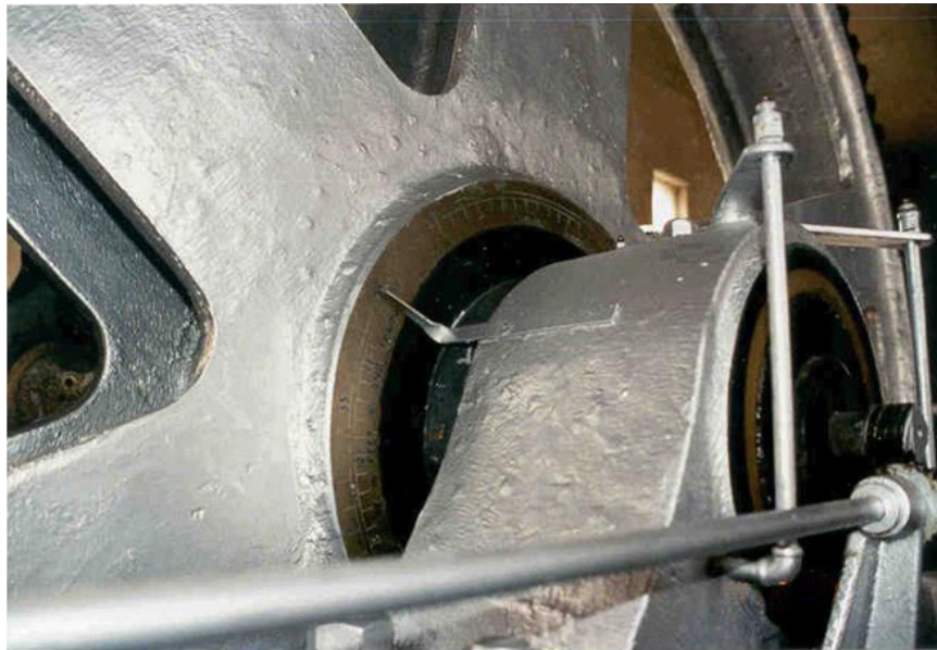
Figure 2-3. Roller Gate Position Indicator
