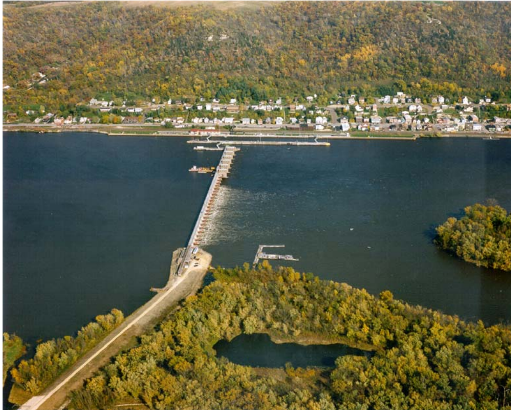
Figure 2-2. Lock and Dam No. 4 (Looking East)
