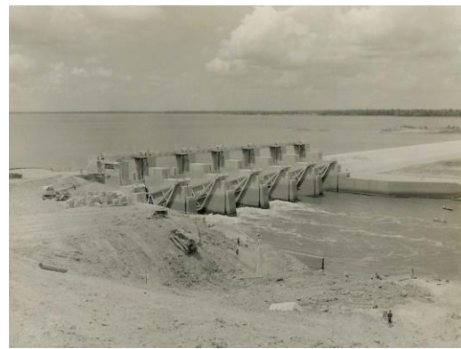
Figure 3-4. Tainter Gates Construction
