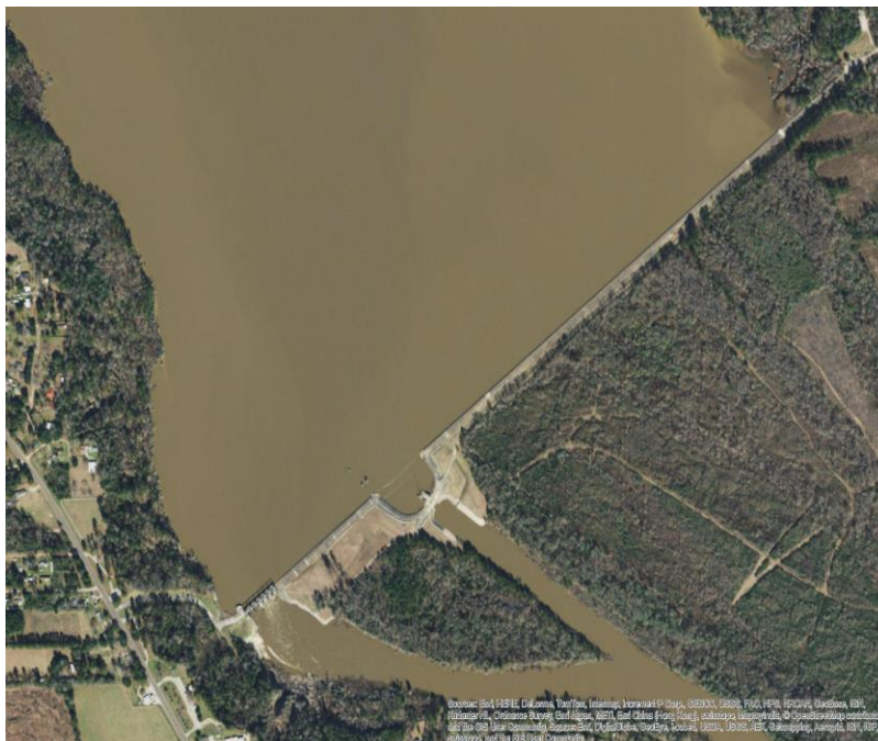
Figure 2-1. Aerial View of Town Bluff Dam
