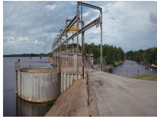
Figure 4-10. 2008 Flood - Lake Elevation near Gated Spillway
