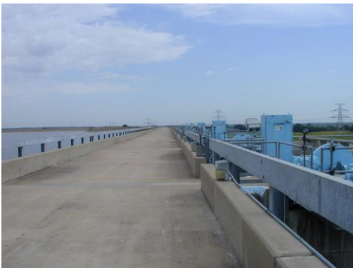
Figure 2-6. Spillway Concrete Road
