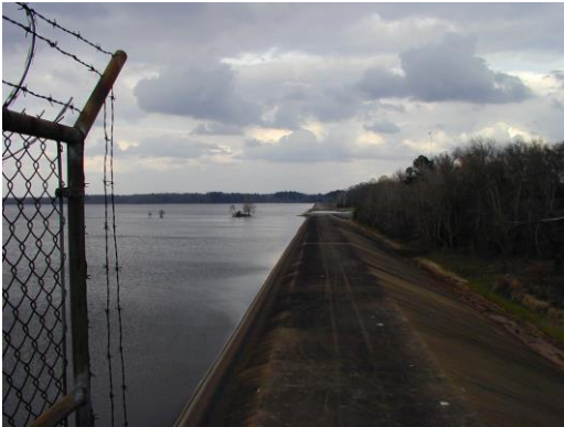
Figure 2-2. Upstream Side of Embankment
