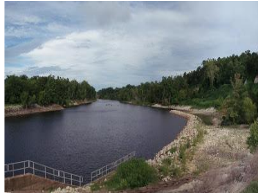
Figure 2-9. Gated Spillway Stilling Basin and Discharge Channel
