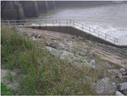
Figure 2-8. Riprap and Concrete Blocks of Gated Spillway
