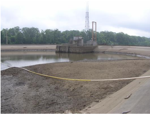
Figure 2-10. Upstream Side of Powerhouse
