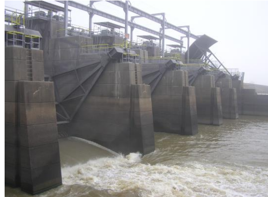
Figure 2-5. Downstream Side of Gated Spillway
