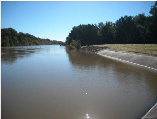
Figure 2-12. Powerhouse Discharge Channel
