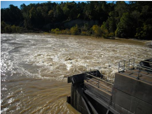
Figure 4-11. 2013 Flood - Downstream of Gated Spillway
