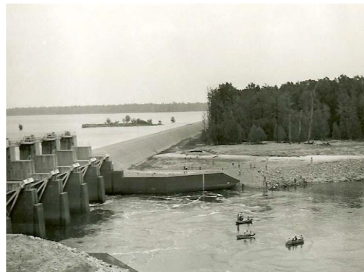
Figure 3-6. Downstream Channel Construction
