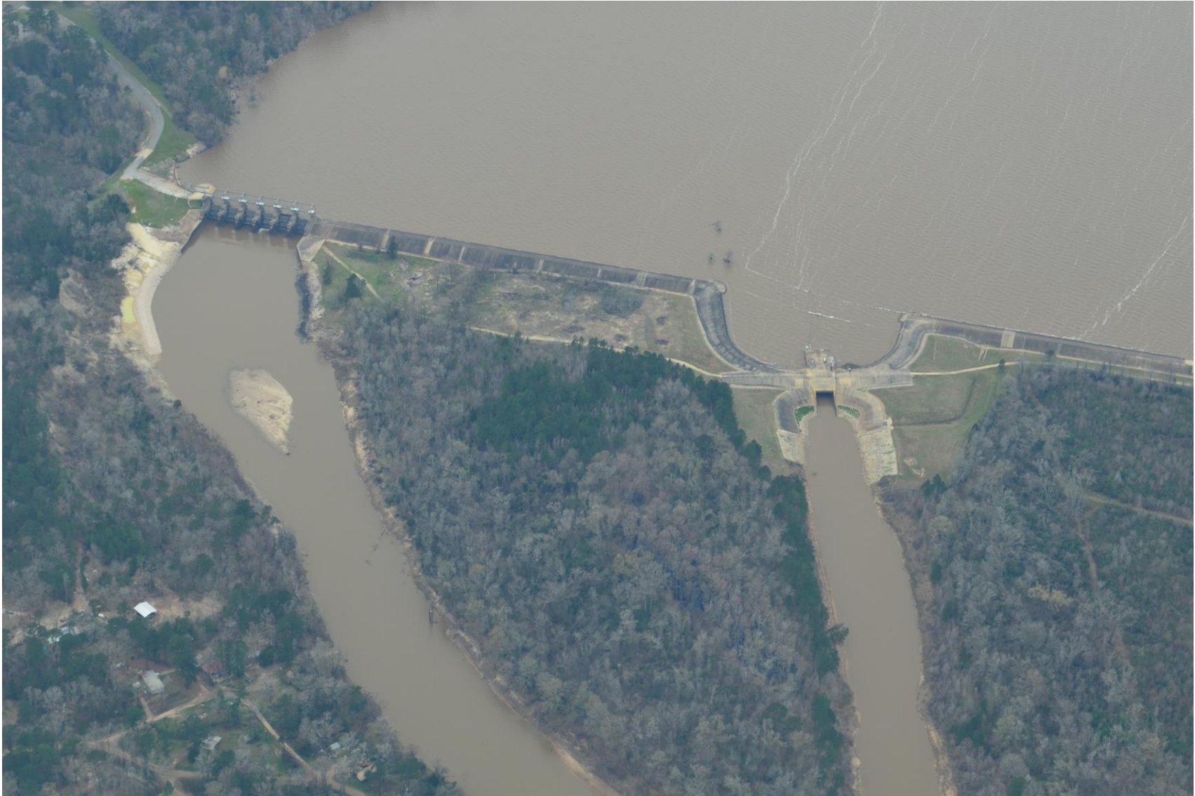
TOWN BLUFF DAM AND B.A. STEINHAGEN LAKE
