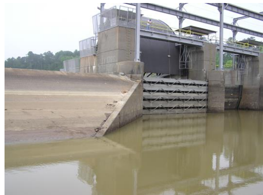
Figure 2-7. Upstream Side of Emergency Stoplog Spillway Gate
