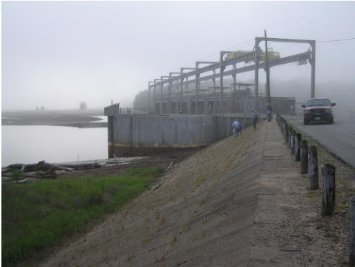
Figure 2-4. Upstream Side of Gated Spillway
