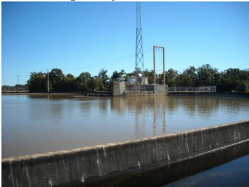
Figure 4-13. 2013 Flood - Upstream of Powerhouse
