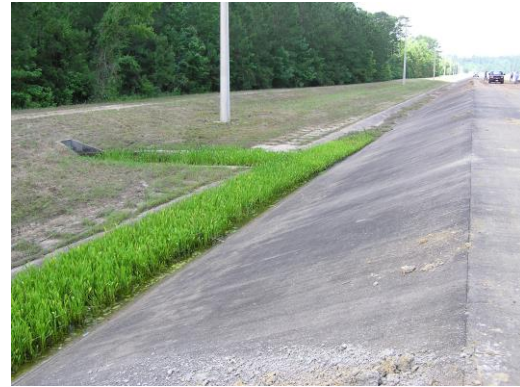
Figure 2-3. Downstream Side of Embankment
