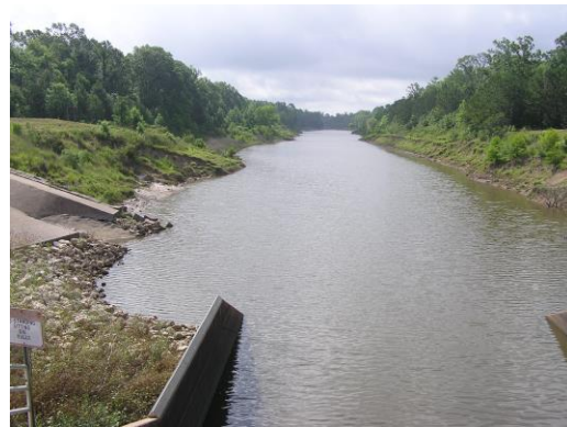
Figure 2-13. Powerhouse Discharge Channel
