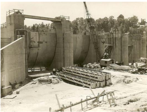
Figure 3-3. Tainter Gates Construction
