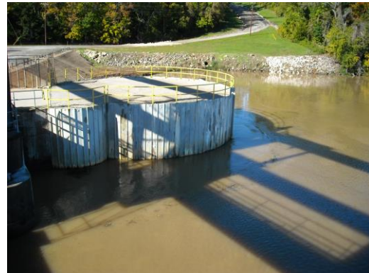
Figure 4-12. 2013 Flood - Upstream of Gated Spillway
