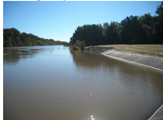
Figure 4-14. 2013 Flood - Powerhouse Discharge Channel
