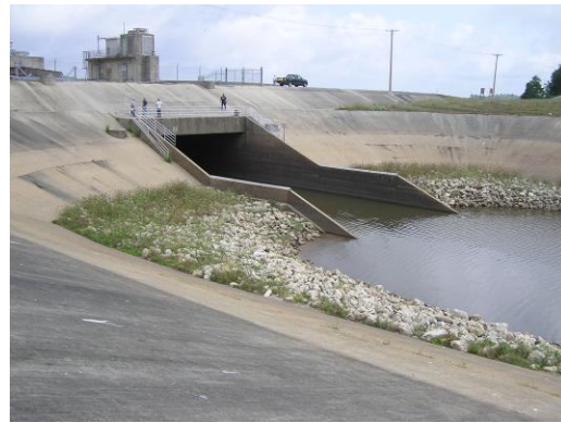
Figure 2-11. Downstream Side of Powerhouse and Stilling Basin
