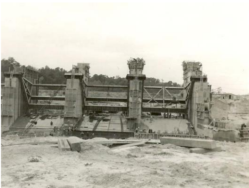
Figure 3-5. Front Structure Construction
