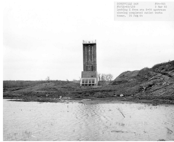
Figure 3-2. View of Intake Structure
