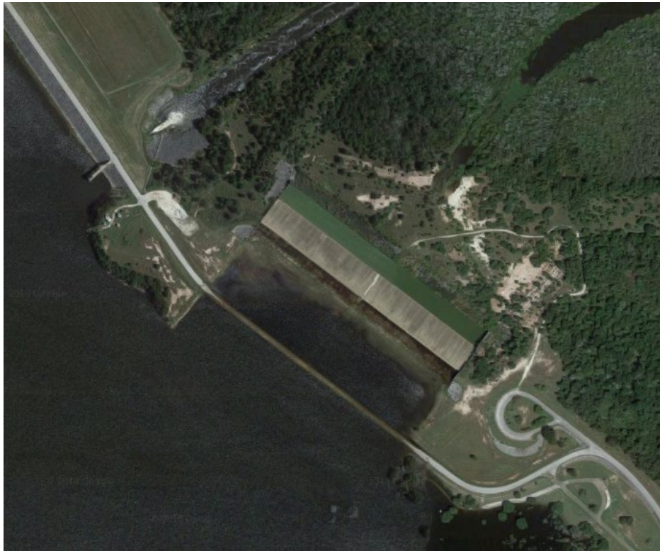
Figure 2-1. Aerial View of Somerville Dam
