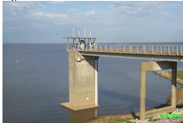
Figure 2-5. Outlet Works Tower
