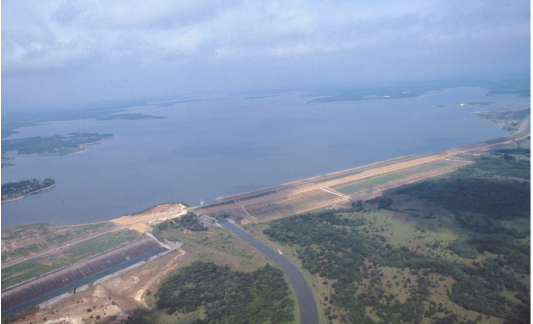
SOMERVILLE DAM AND LAKE
