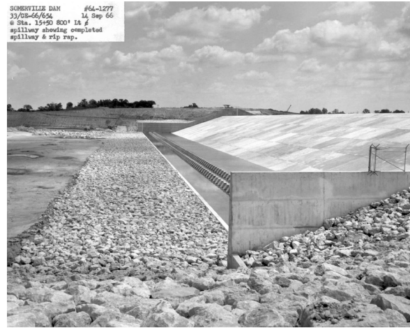
Figure 3-8. Profile View: Completed Spillway, Riprap and Baffling Blocks
