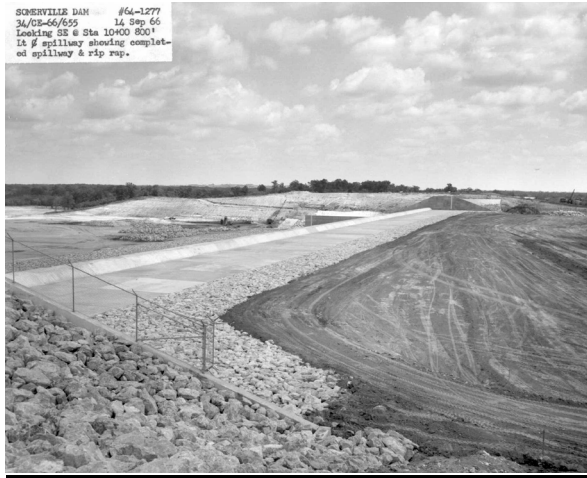
Figure 3-7. Completed Spillway and Riprap
