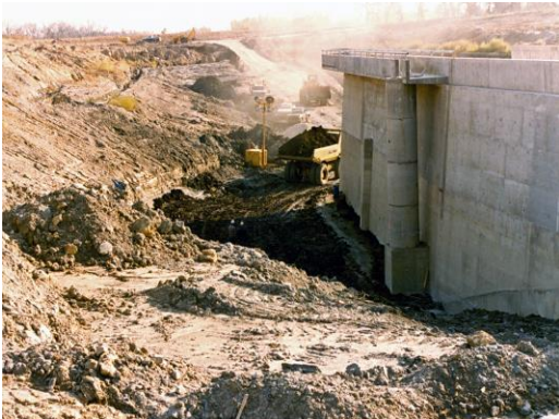
Figure 3-1. Dam Construction – Outlet Works
