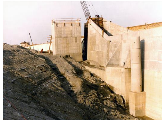
Figure 3-2. Dam Construction – Outlet Works
