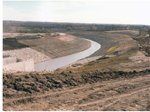
Figure 3-6. Dam Construction – Discharge Channel
