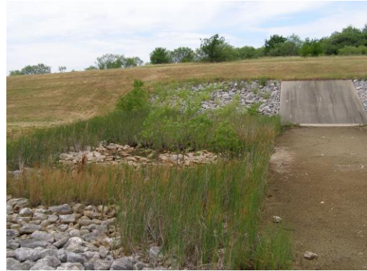
Figure 2-5. Spillway Concrete Sill and Riprap
