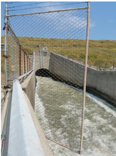
Figure 2-10. Discharge Tunnel and Stilling Basin
