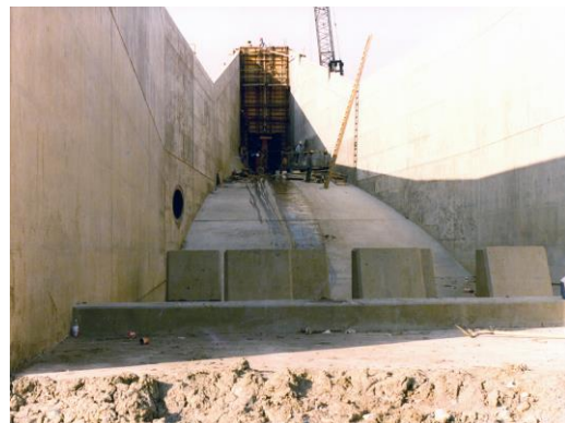
Figure 3-4. Dam Construction – Outlet Works
