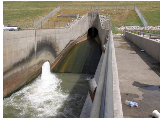
Figure 2-9. Outlet Conduit and 5-foot diameter Low Flow Conduit
