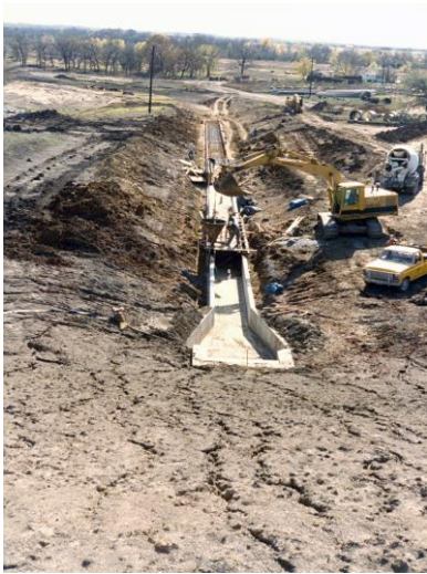
Figure 3-7. Dam Construction – Discharge Channel
