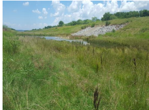
Figure 2-7. Spillway Concrete Sill and Riprap
