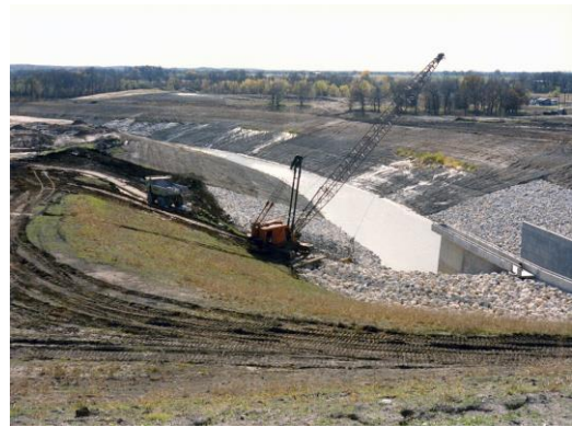
Figure 3-8. Dam Construction – Discharge Channel
