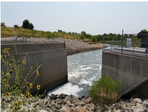
Figure 2-12 Retaining Wall and Powerhouse Platform
