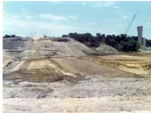
Figure 3-2. Embankment Fill Operations
