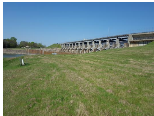
Figure 2-3. Downstream View of Embankment
