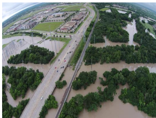
Figure 4-7. 2015 Flood - Flooded Area around Highway 78
