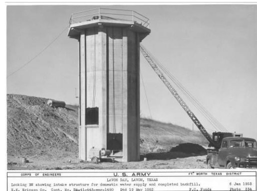
Figure 3-10. Dam Construction - Intake Structure
