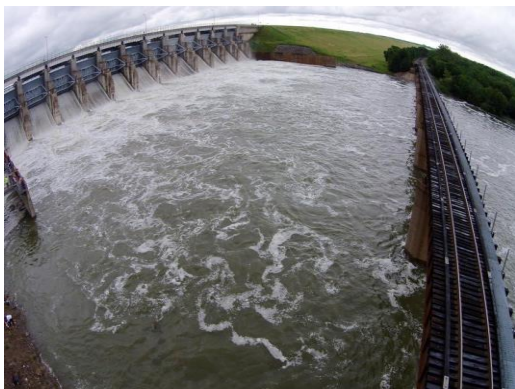
Figure 4-2. 2015 Flood - Water Released from Spillway
