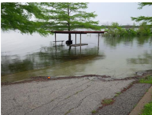
Figure 4-6. 2015 Flood - Inundated Pavilion
