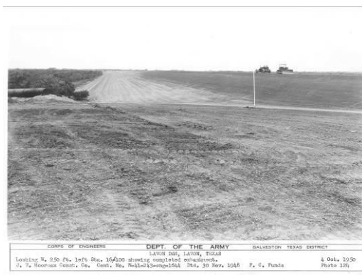
Figure 3-3. Dam Construction - Embankment
