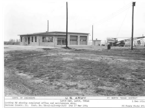
Figure 3-12. Dam Construction - Office and Maintenance Shop
