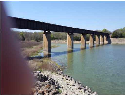
Figure 2-8. Train Bridge Downstream of Spillway
