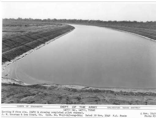
Figure 3-1. Dam Construction - Pilot Channel
