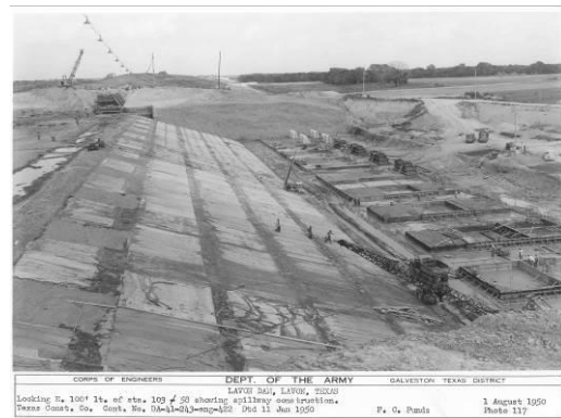
Figure 3-2. Dam Construction - Spillway
