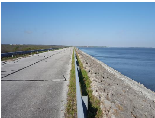
Figure 2-2. Upstream View of Embankment
