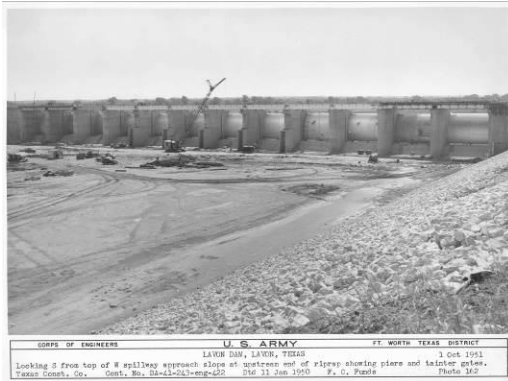
Figure 3-7. Dam Construction - Piers and Tainter Gates
