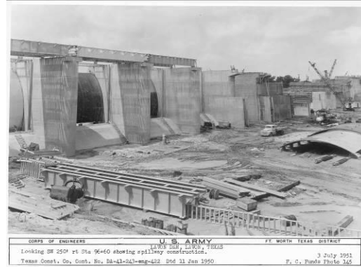
Figure 3-6. Dam Construction - Spillway
