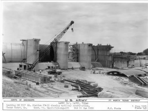
Figure 3-5. Dam Construction - Spillway
