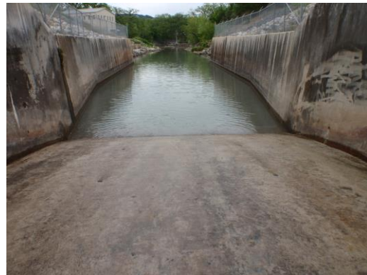
Figure 2-11. Outlet Discharge Tunnel
