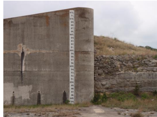
Figure 2-7. Spillway Retaining Wall
