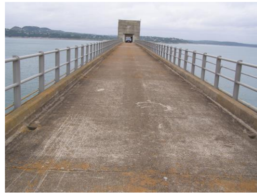
Figure 2-9. Intake Tower and Access Bridge
