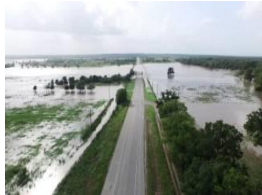
Figure 4-16. 2015 Flood - Guadalupe River
