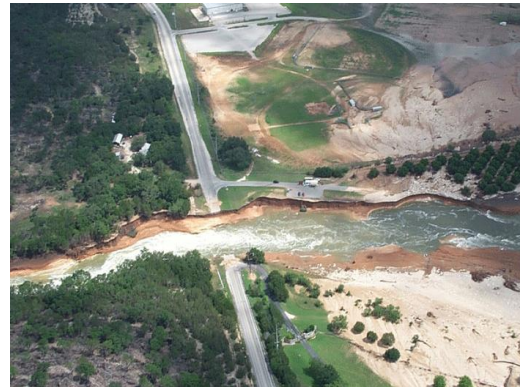
Figure 4-6. 2002 Flood - Access Road Downstream Discharge Channel
