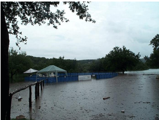
Figure 4-7. 2002 Flood - Park Area
