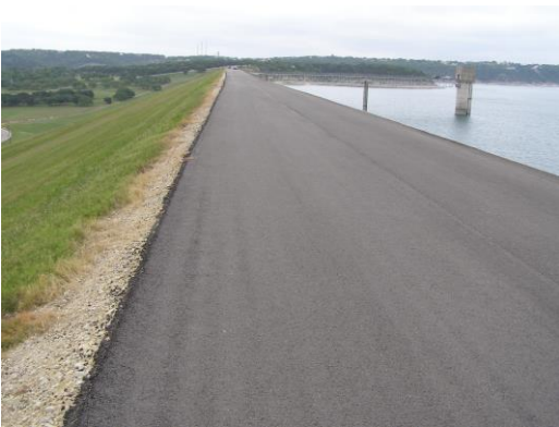
Figure 2-4. Dam Road and Downstream View of Embankment
