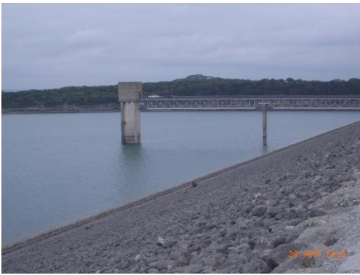
Figure 2-2. Upstream View of Embankment and Intake Tower
