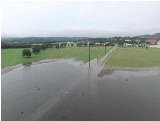
Figure 4-13. 2015 Flood - Marina Access Road
