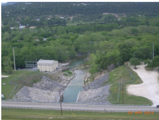
Figure 2-12. Stilling Basin and Discharge Channel
