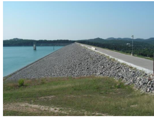
Figure 2-3. Upstream View of Embankment
