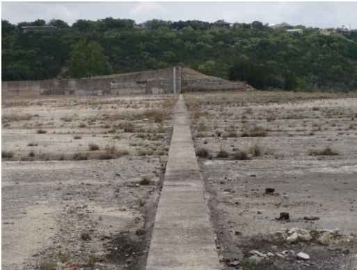
Figure 2-6. Crest of Spillway
