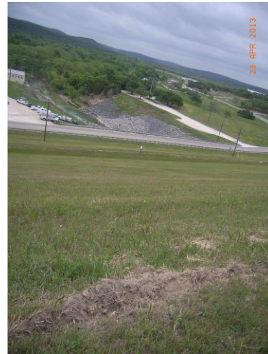
Figure 2-5. Downstream View of Embankment
