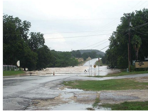
Figure 4-10. 2002 Flood - Access Road
