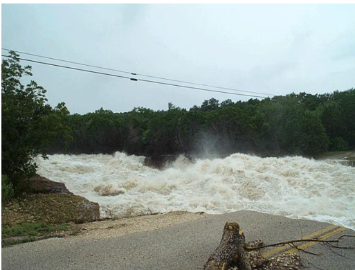
Figure 4-11. 2002 Flood - Access Road
