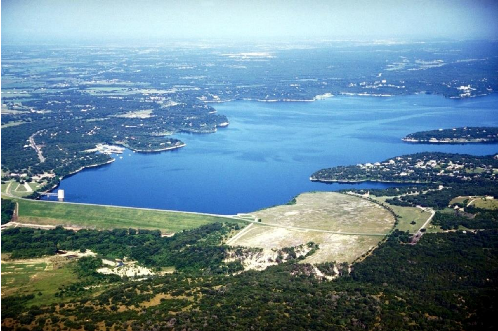
BELTON DAM AND LAKE
