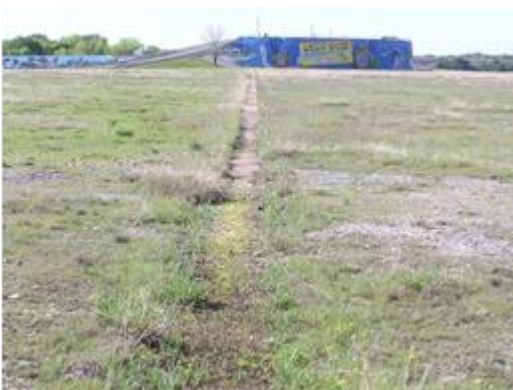
Figure 2-4. Top of Spillway
