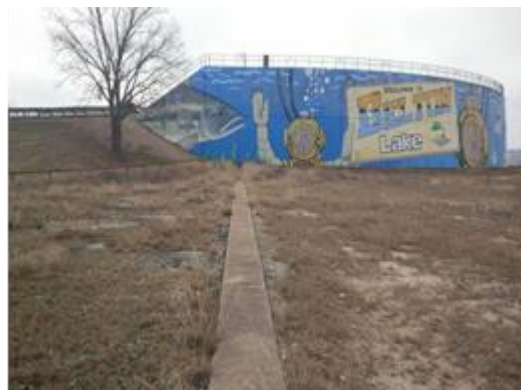
Figure 2-5. Spillway Sill and Training Wall
