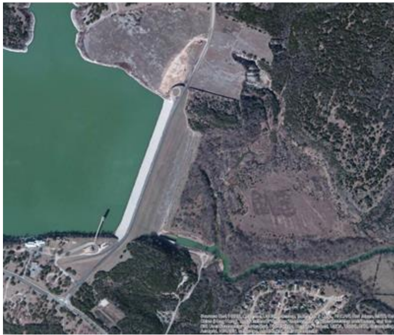
Figure 2-1. Aerial View of Belton Dam
