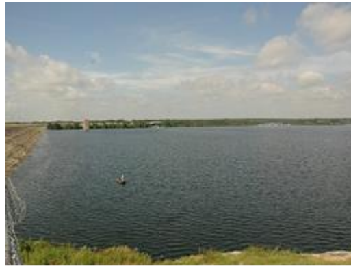
Figure 4-3. Lake Elevation near Embankment
