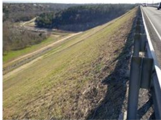
Figure 2-3. Downstream View of Embankment
