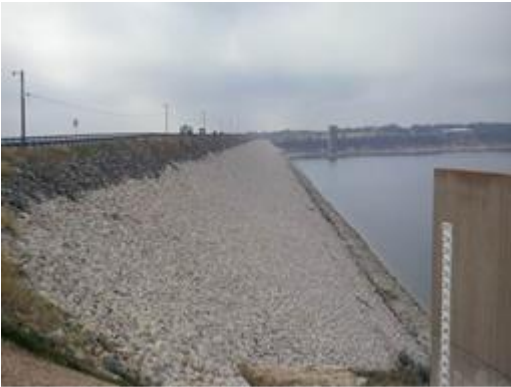
Figure 2-2. Upstream View of Embankment
