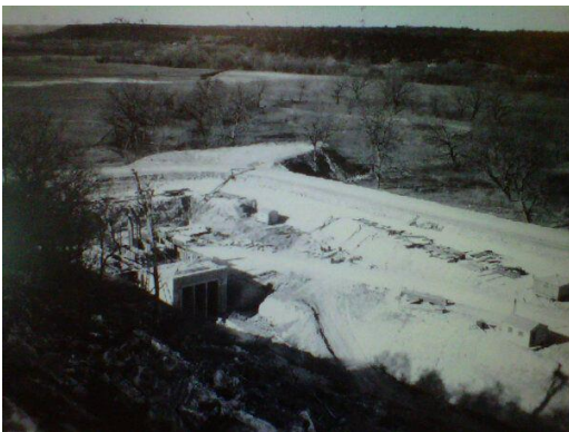
Figure 3-3. Construction of Floodgates on Spillway Side, 1952
