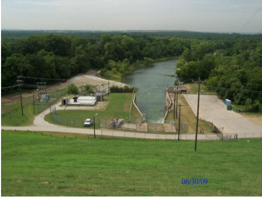
Figure 2-12. Stilling Basin and Discharge Channel
