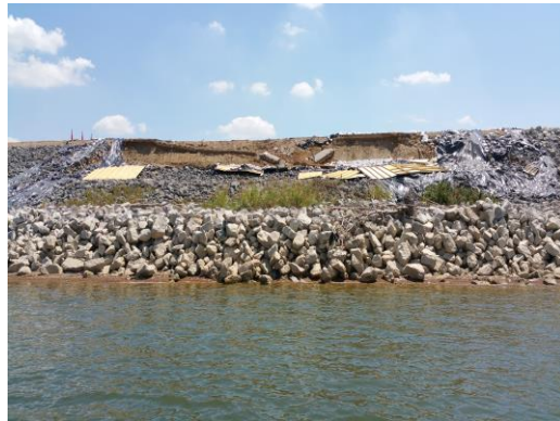
Figure 2-5. Embankment Slide of August 2015 Flood
