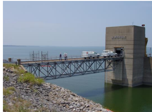
Figure 2-9. Intake Tower and Access Bridge
