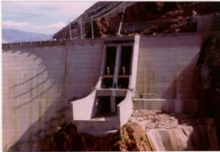
Photo 2-3. Modified Roosevelt Dam - Left Spillway Structure
