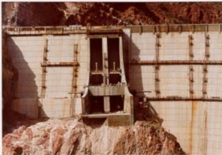
Photo 2-4. Modified Roosevelt Dam - Right Spillway Structure
