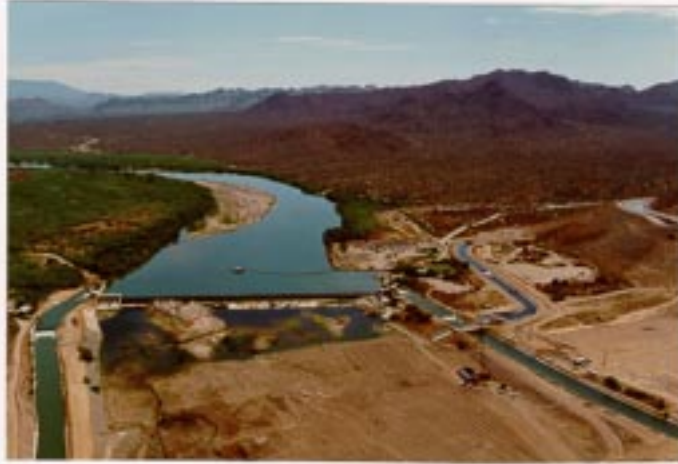
Photo 2-9. Granite Reef Diversion Dam
