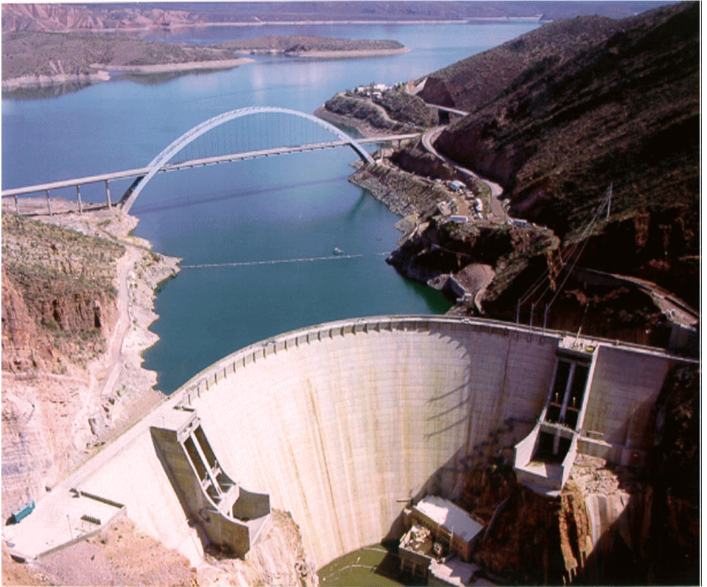
Aerial Photograph of Modified Roosevelt Dam and Theodore Roosevelt Lake
