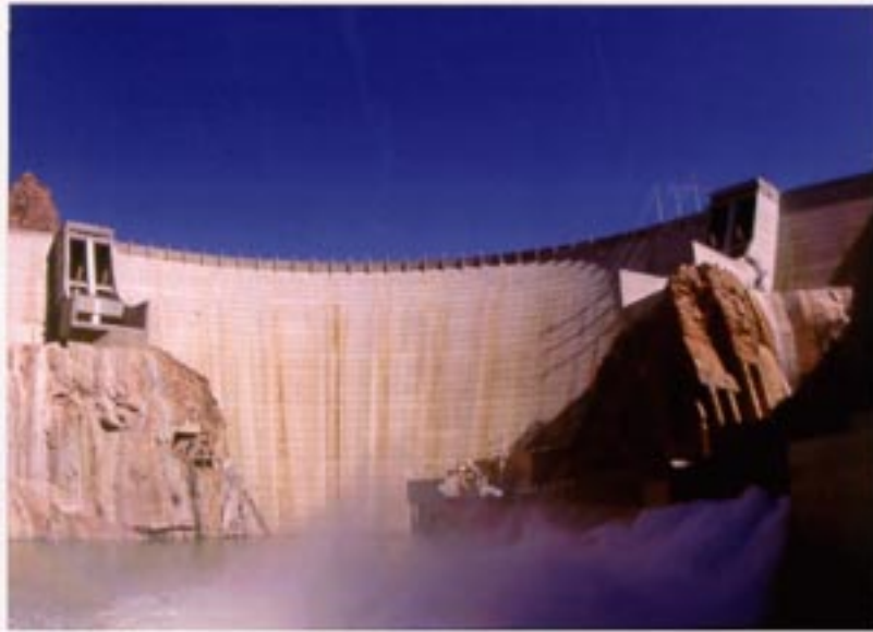
Photo 2-1. Modified Roosevelt Dam - Upstream View.
