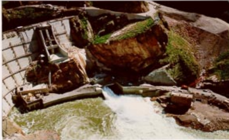
Photo 2-7. Modified Roosevelt Dam - River Outlet Works
