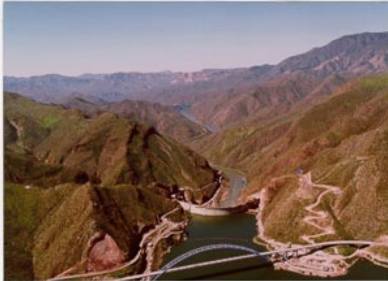
Photo 2-2. Modified Roosevelt Dam - Downstream View
