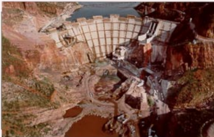
Photo 2-5. Modified Roosevelt Dam - Plunge Pool Area
