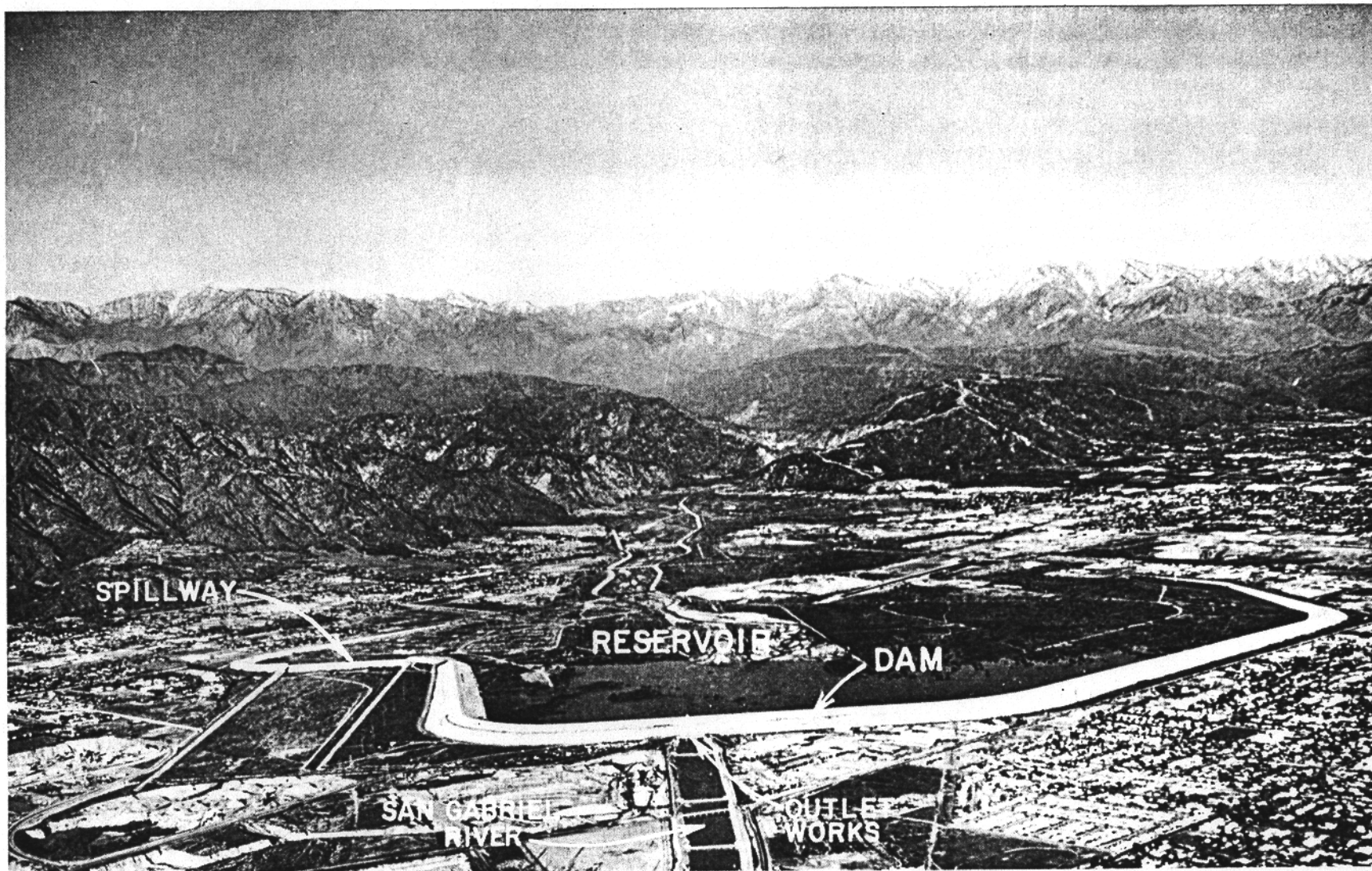
SANTA FE DAM AND RESERVOIR
