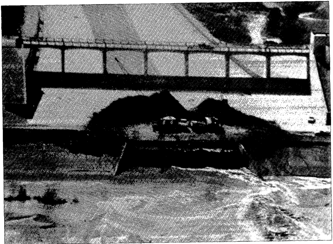
Figure 3-4. Debris at Hansen Dam after March 1, 1983 storm.
