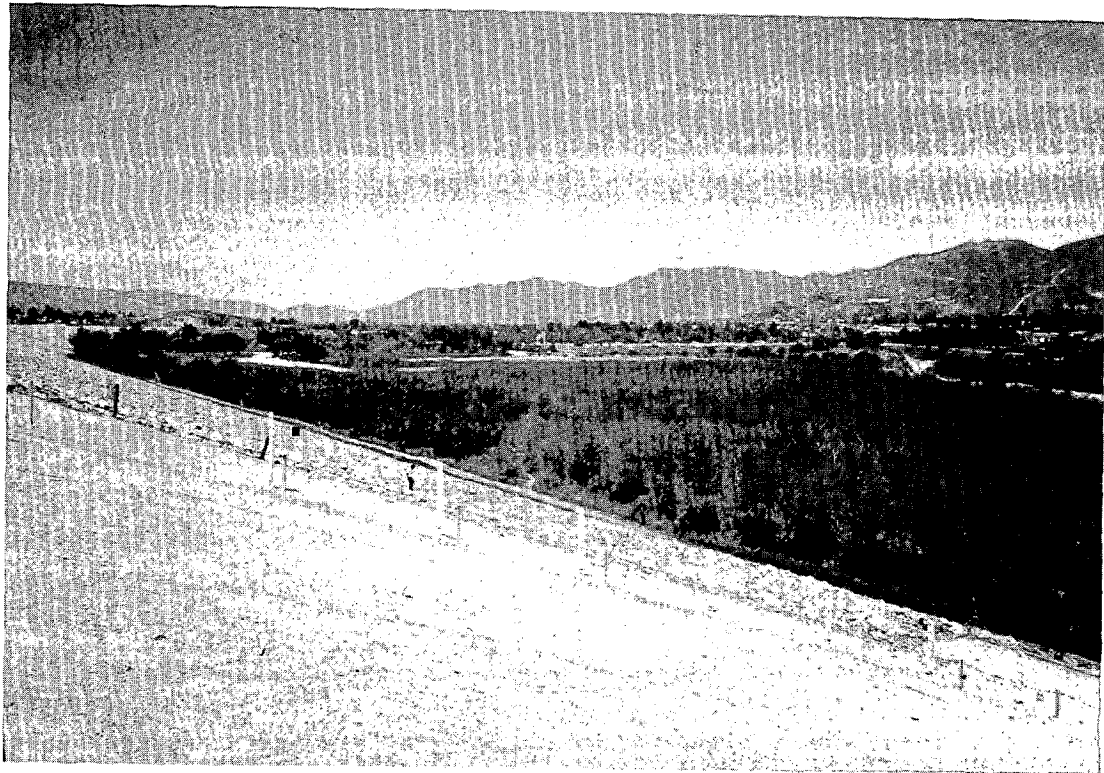
Figure 2-1b. Upstream View of Hansen Dam Embankment, Looking Northwest
