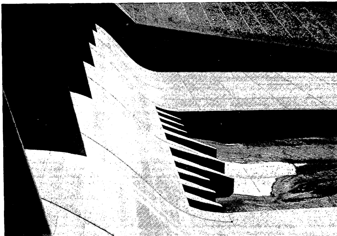
Figure 2-3. Hansen Dam Spillway and Outlet Channel.
