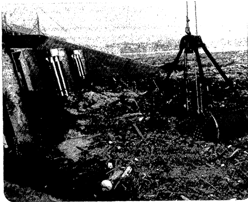
Figure 3-3. Debris at Hansen Dam after February 17, 1980 storm.
