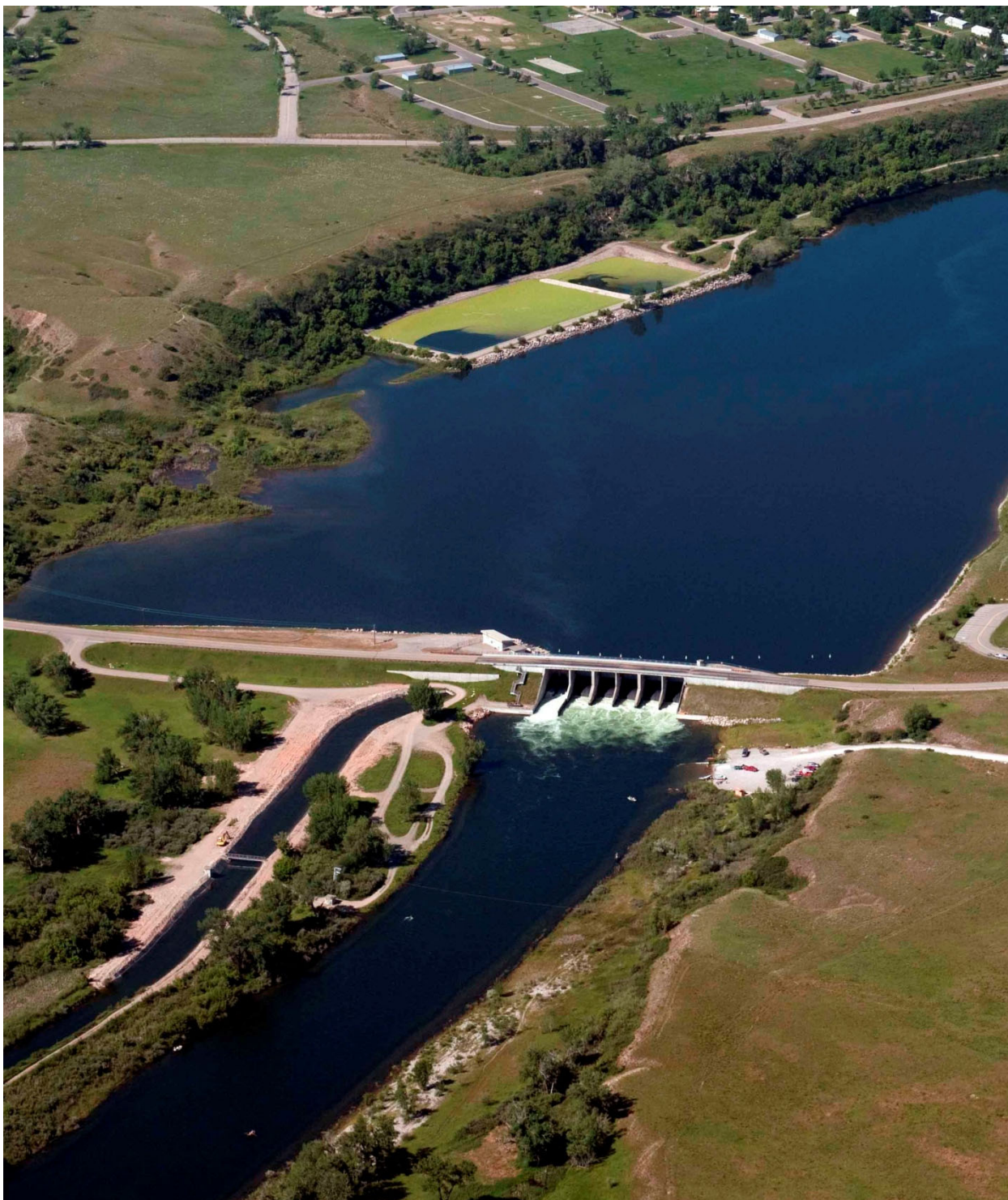
Yellowtail's Afterbay Dam and Bighorn Canal
