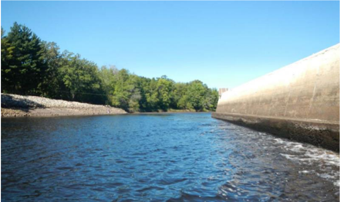
Figure 4-13. General View of Downstream Channel
