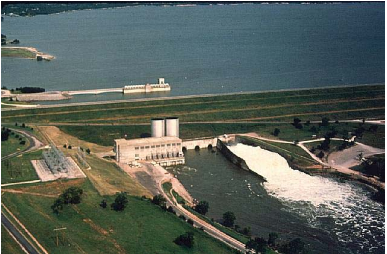
POWERHOUSE, OUTLET WORKS, AND DAM AT LAKE TEXOMA (DENISON DAM)
