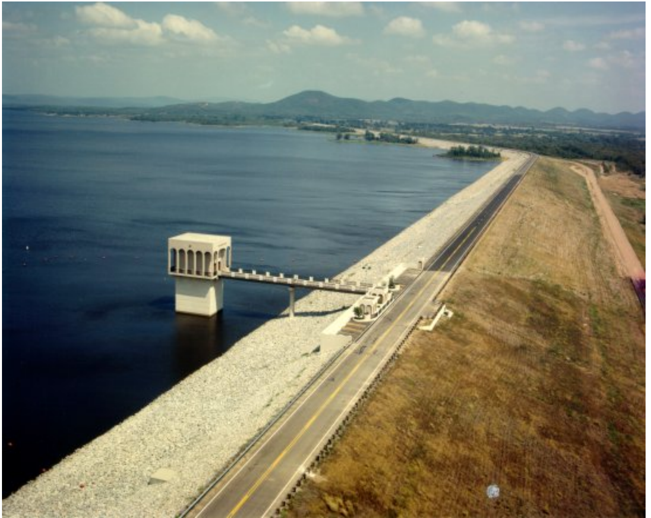
LOOKING NORTHEAST AT SARDIS DAM EMBANKMENT AND OUTLET WORKS TOWER
