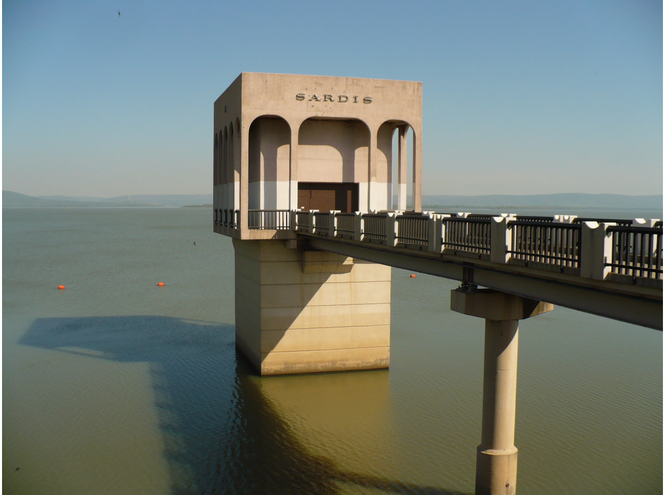
OUTLET WORKS TOWER AT SARDIS LAKE
