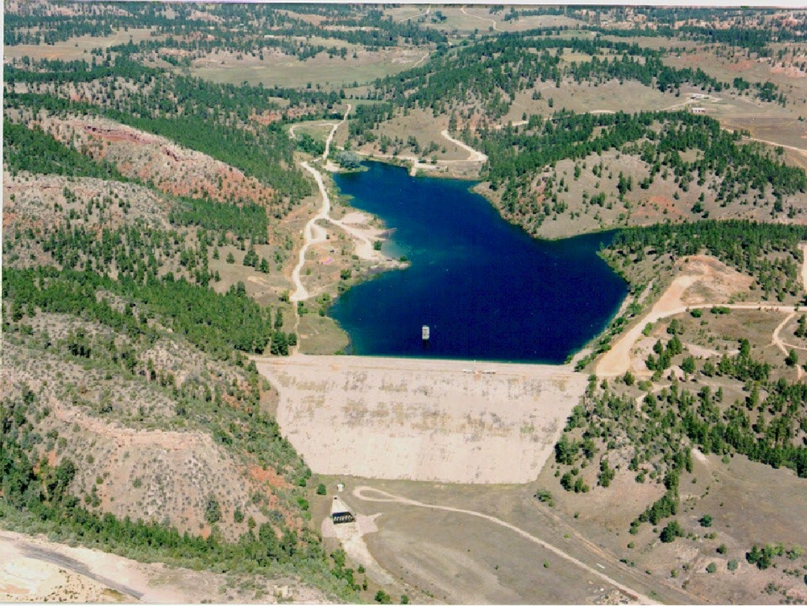
Figure 1-1 Cold Brook Dam and Reservoir (looking northwest)
