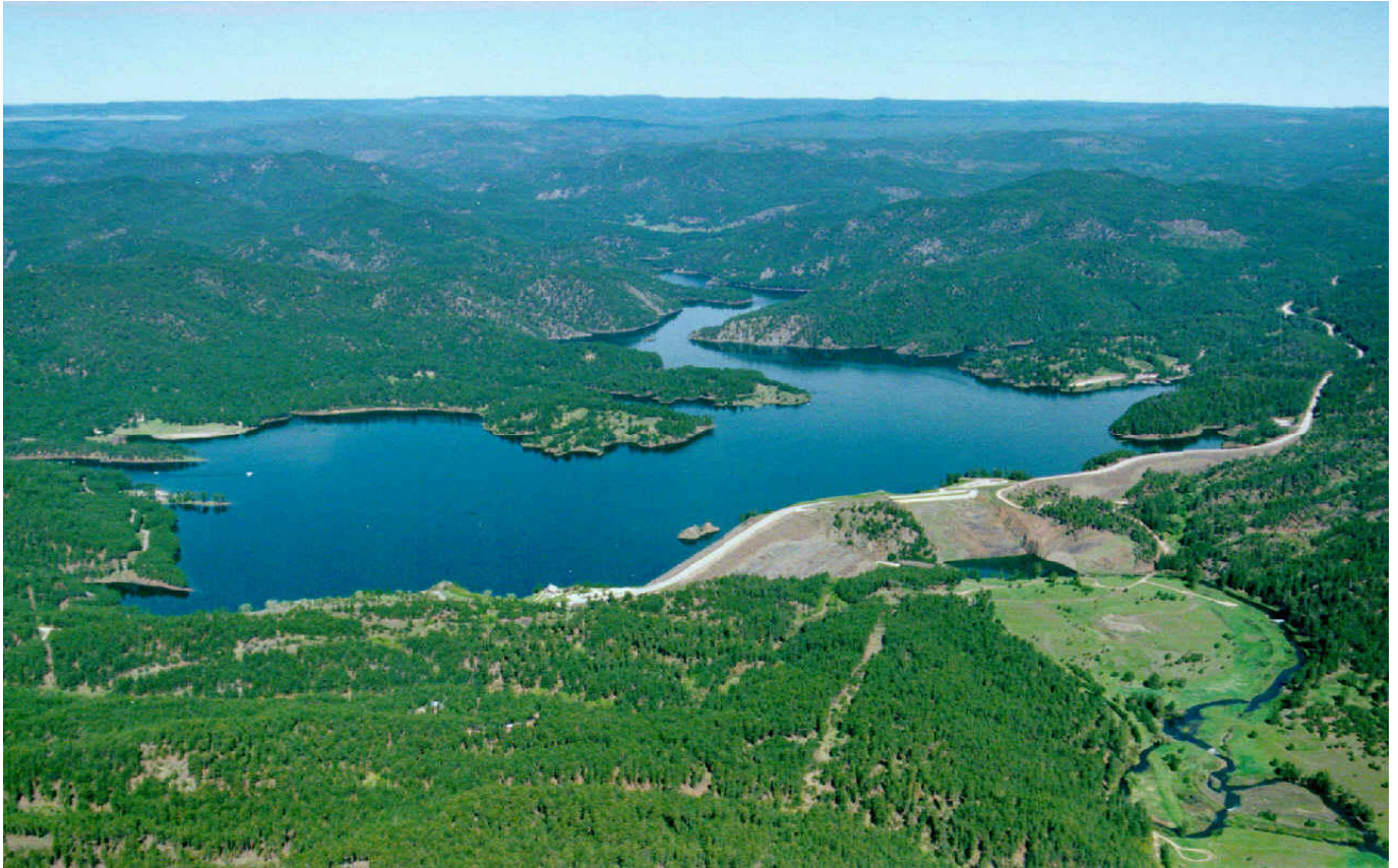
Figure 1-1 Pactola Dam and Reservoir
