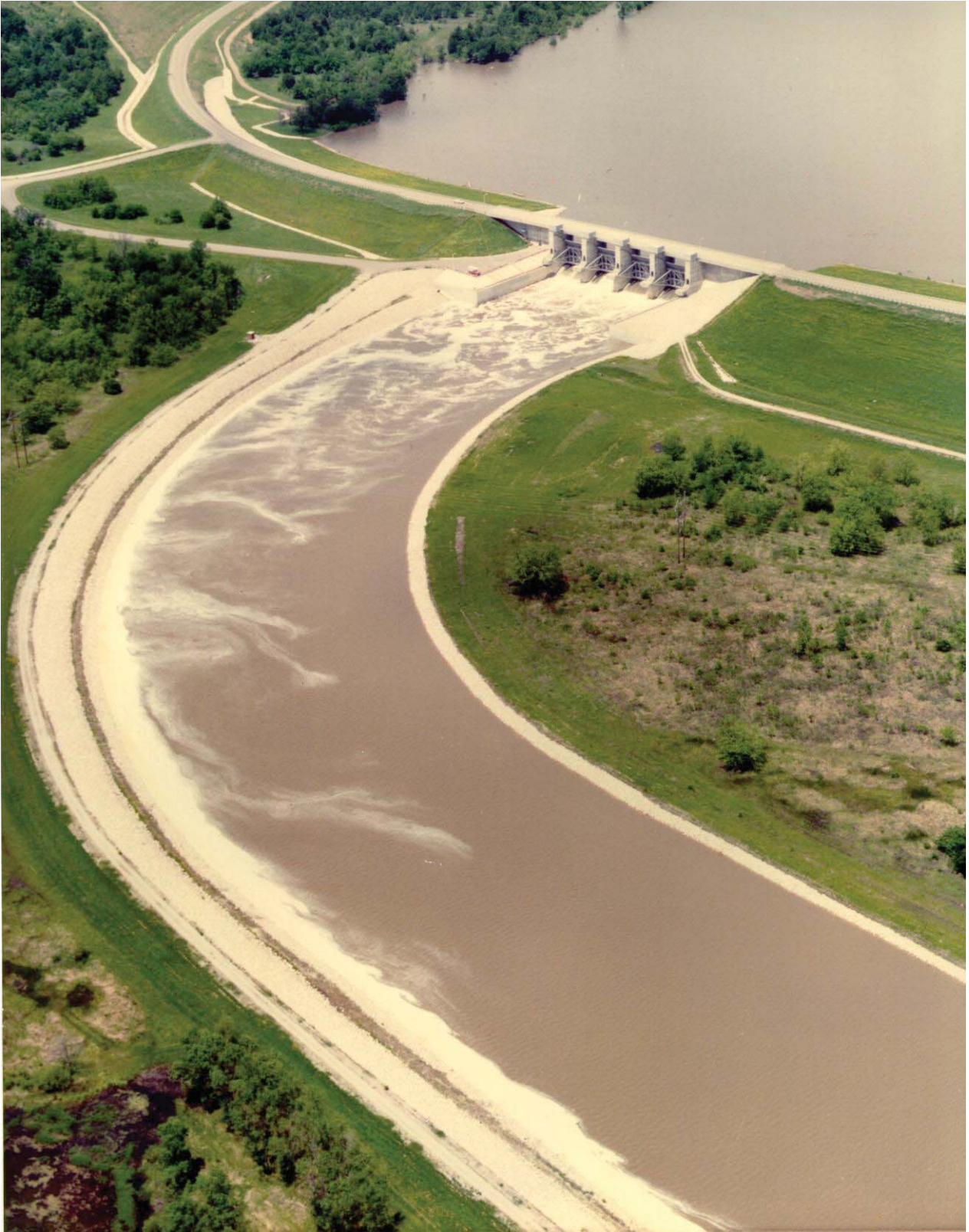
LOOKING NORTH AT COPAN DAM AND TAITNER GATES
