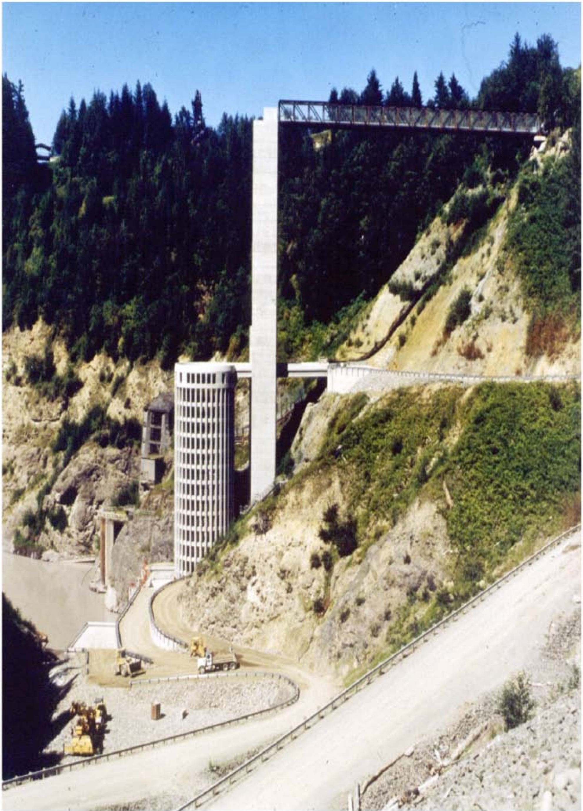
MUD MOUNTAIN DAM INTAKE STRUCTURE
