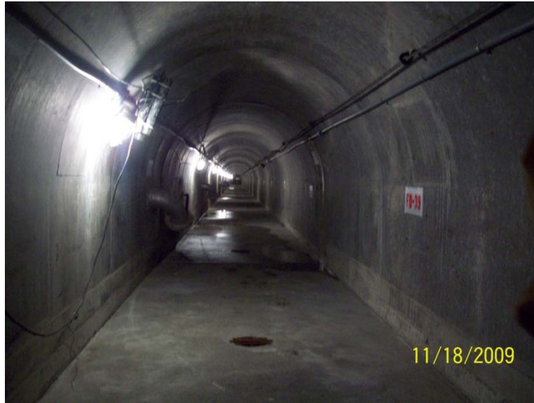
Figure 2-11. Interior view of drainage tunnel.
