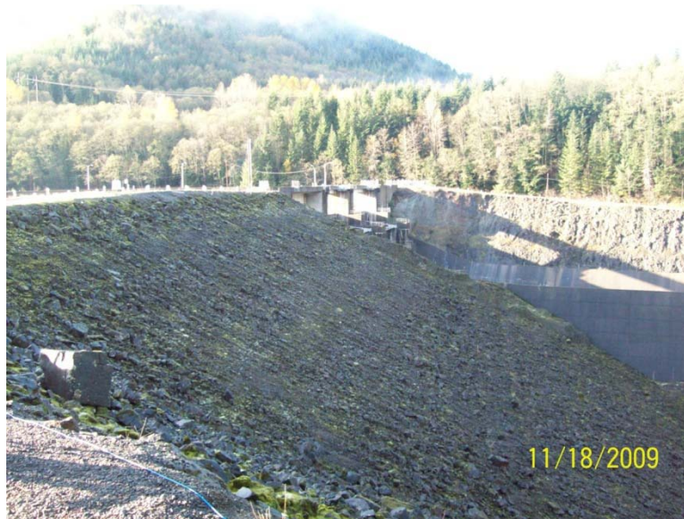
Figure 2-1. Downstream side of embankment dam.
