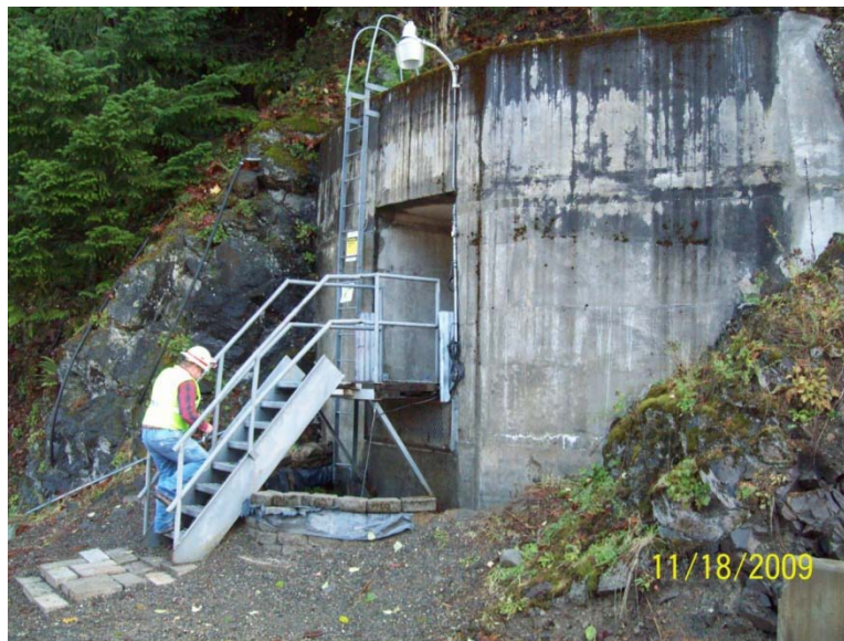
Figure 2-10. Drainage tunnel outlet.
