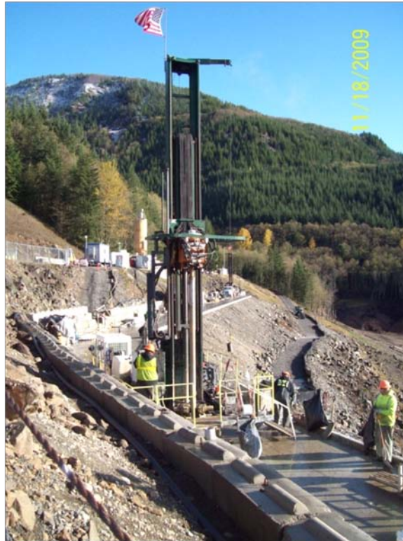
Figure 2-13. Grout injection along right abutment.
