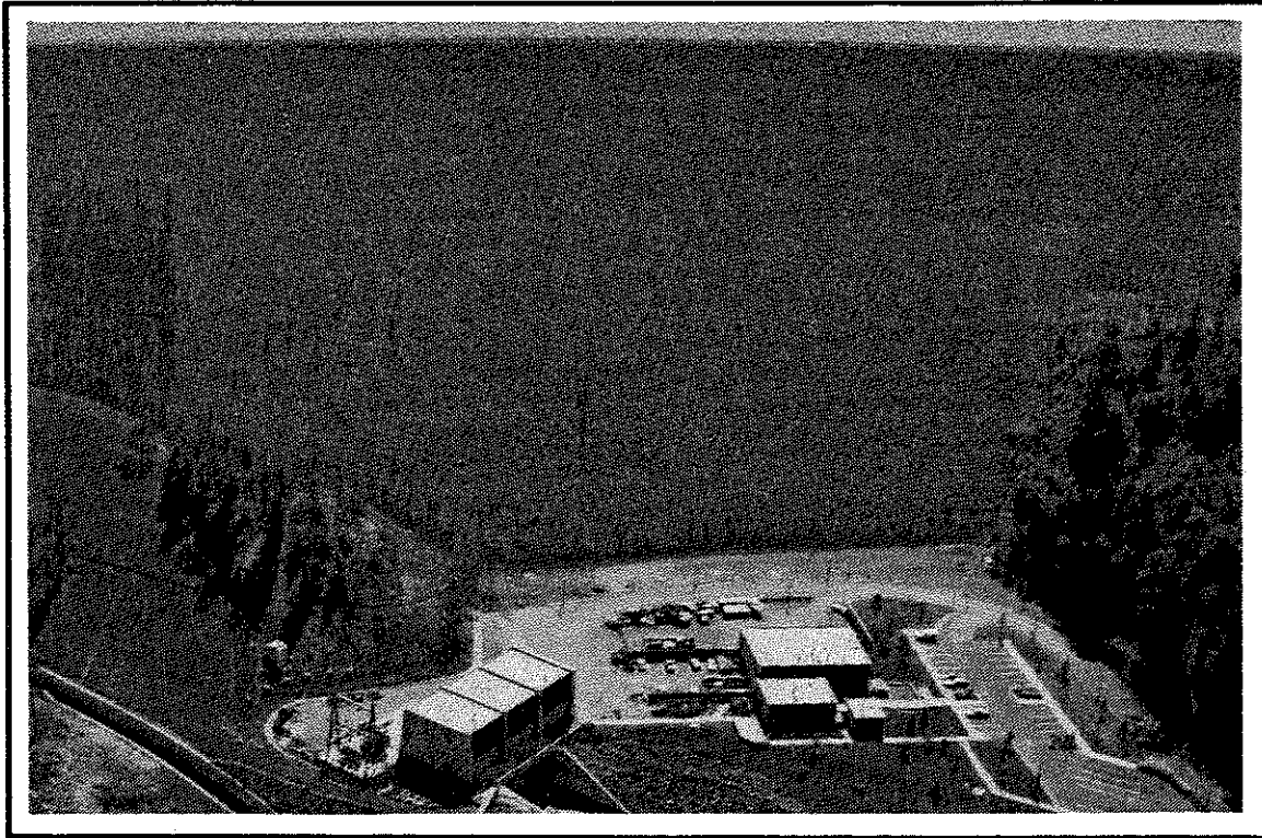
Embankment at Lost Creek Lake
