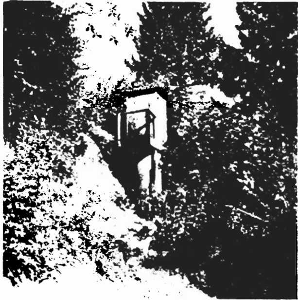
CASCADIA, INFLOW GAGING STATION
