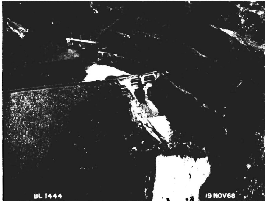
SPILLWAY IN OPERATION (SPECIAL SITUATION)
