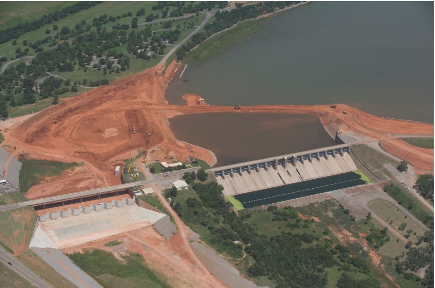
Canton Dam, Service Spillway, and Auxiliary Spillway
