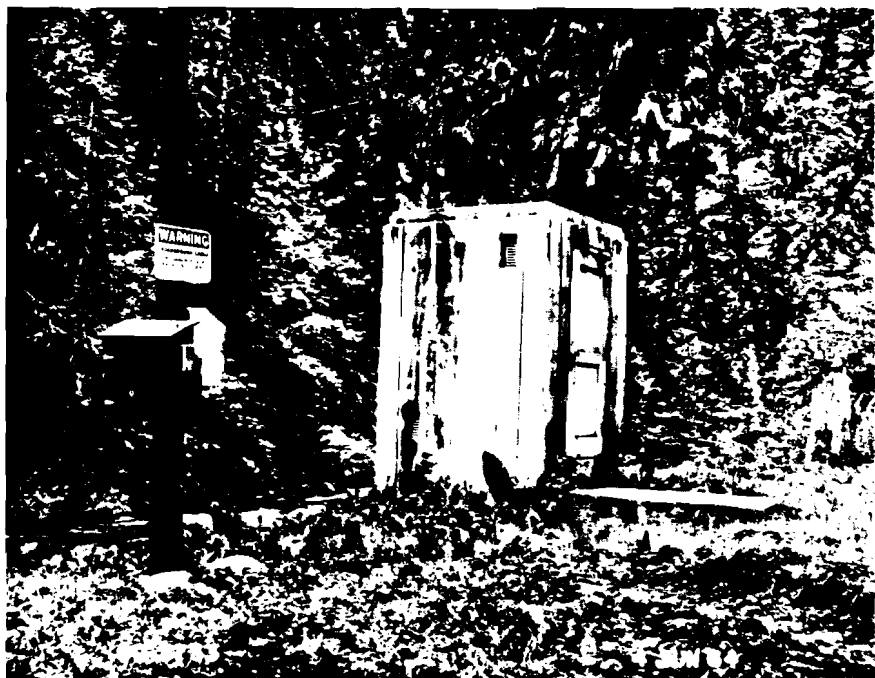
UPSTREAM GAGING STATION South Fork McKenzie River above Cougar Reservoir, near Rainbow, Oregon
