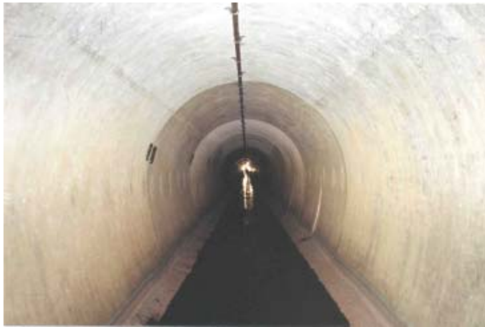
Figure 2-3. Steel-Lined Horseshoe Conduit
