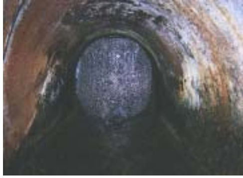
Figure 2-4. 48-inch Steel Conduit Looking at Slide Gate
