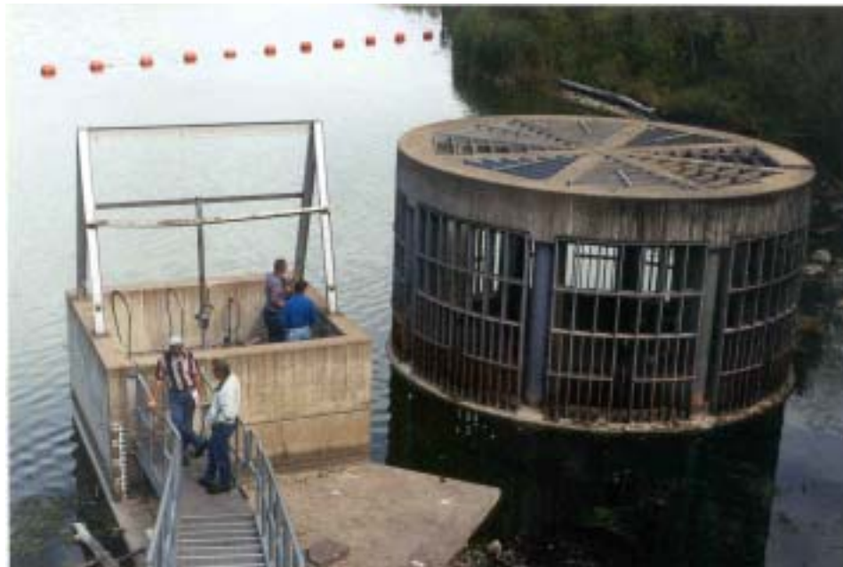
Figure 2-6. Control Tower for Low Flow Inlet
