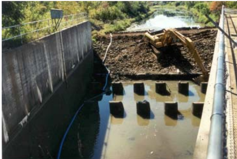
Figure 2-7. Stilling Basin During Periodic Inspection
