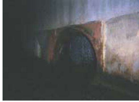
Figure 2-5. Low Flow Inlet to the Horseshoe Conduit
