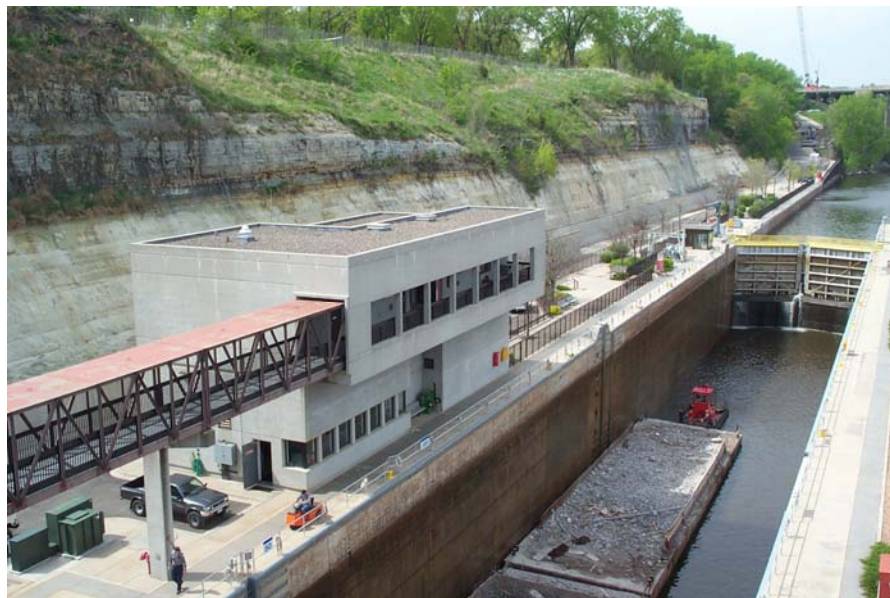
Figure 2-5. Lock and Dam No. 1 Visitor Center.
