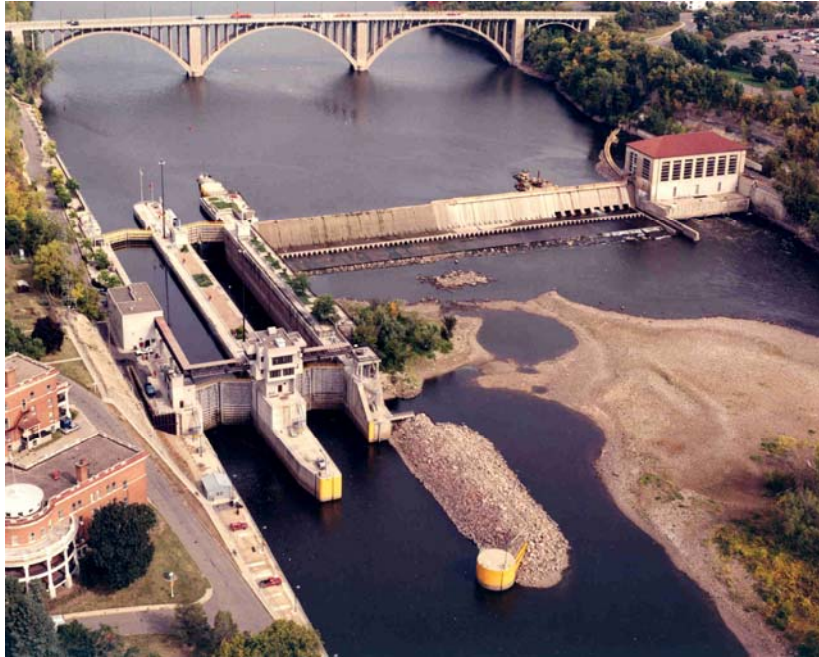
Figure 2-1. Lock and Dam No. 1 – 1996
