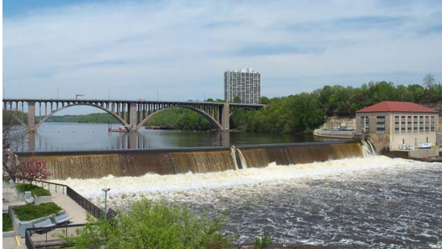
Figure 2-3. Dam and Powerhouse. Bladders Inflated.
