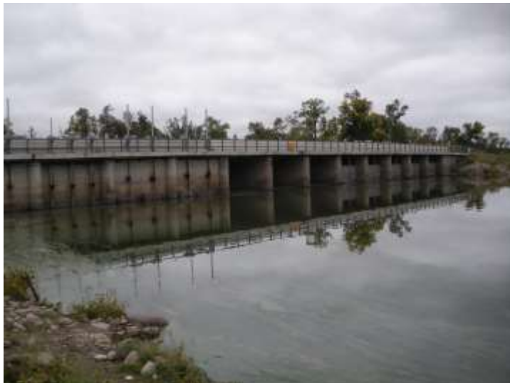
Looking at the upstream side of the Dam.
