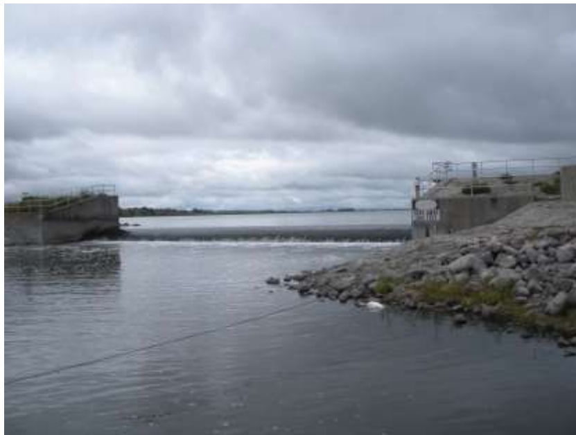
Marsh Lake Dam Looking Upstream (Photos will be updated once project is complete)
