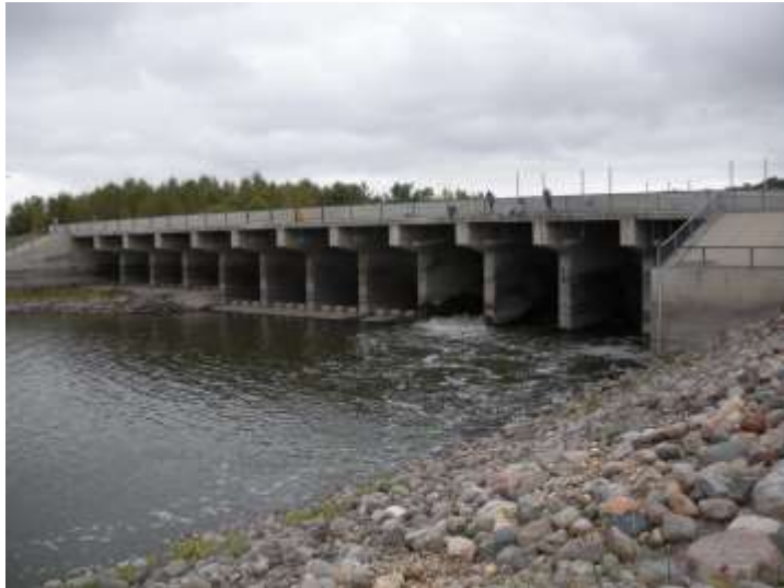
Looking at the downstream side of the Dam.
