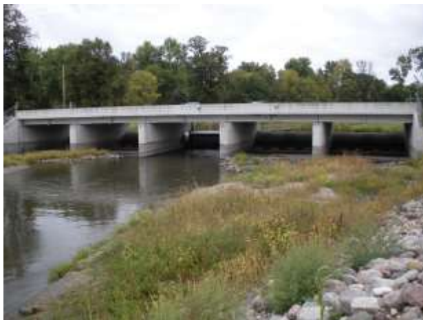
Chippewa Diversion Dam
