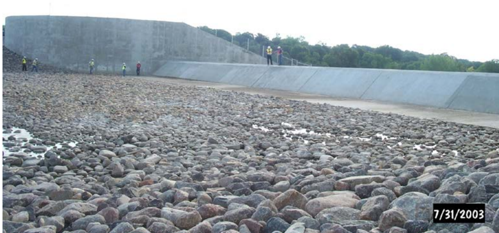
Figure 2-3. Approach Channel to the Spillway.
