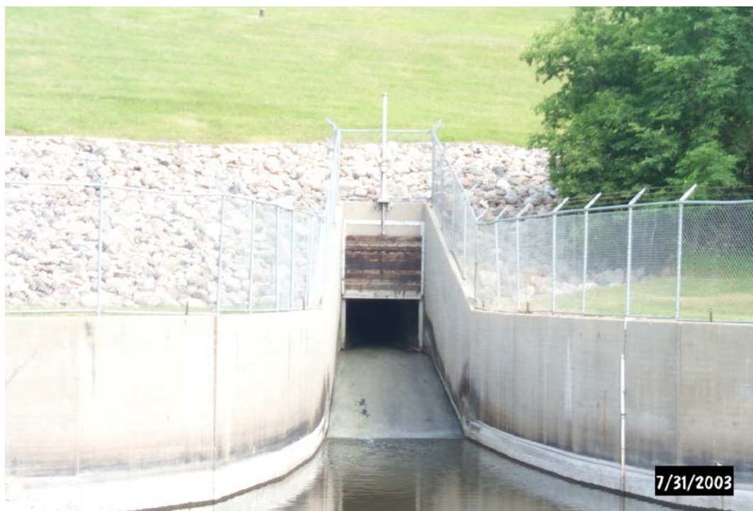
Figure 2-7. Low Flow Outlet.
