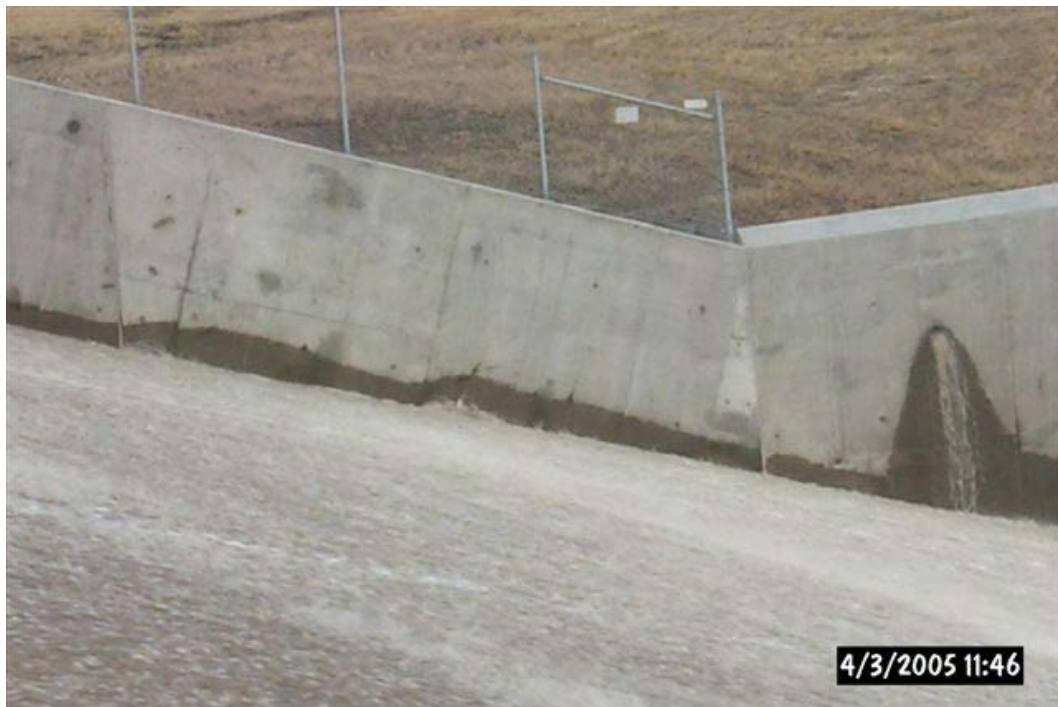
Figure 3-1. Flow Through a Spillway Drain.
