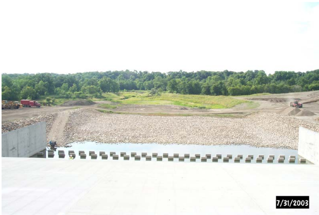
Figure 2-5. Homme Dam Stilling Basin and Outlet Channel.
