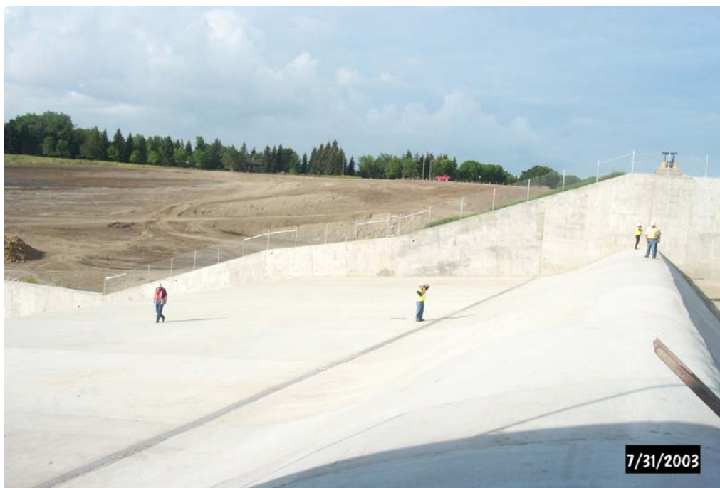
Figure 2-4. Homme Dam Spillway.
