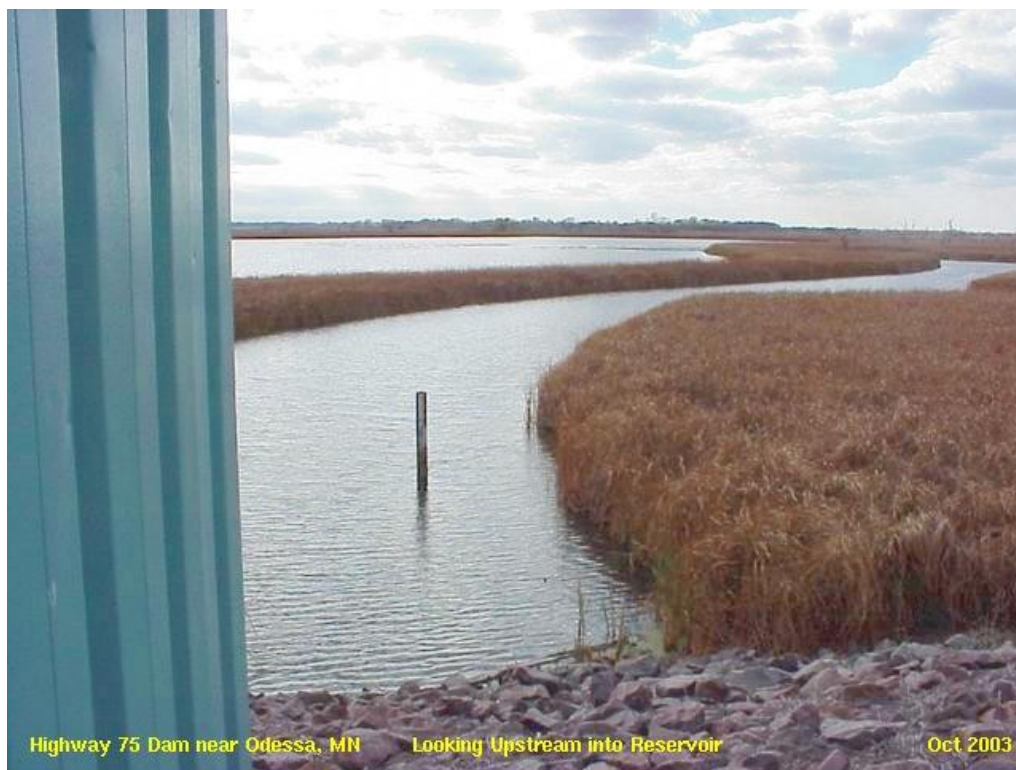
Figure 2-3. Low Flow Channel - Looking Upstream.
