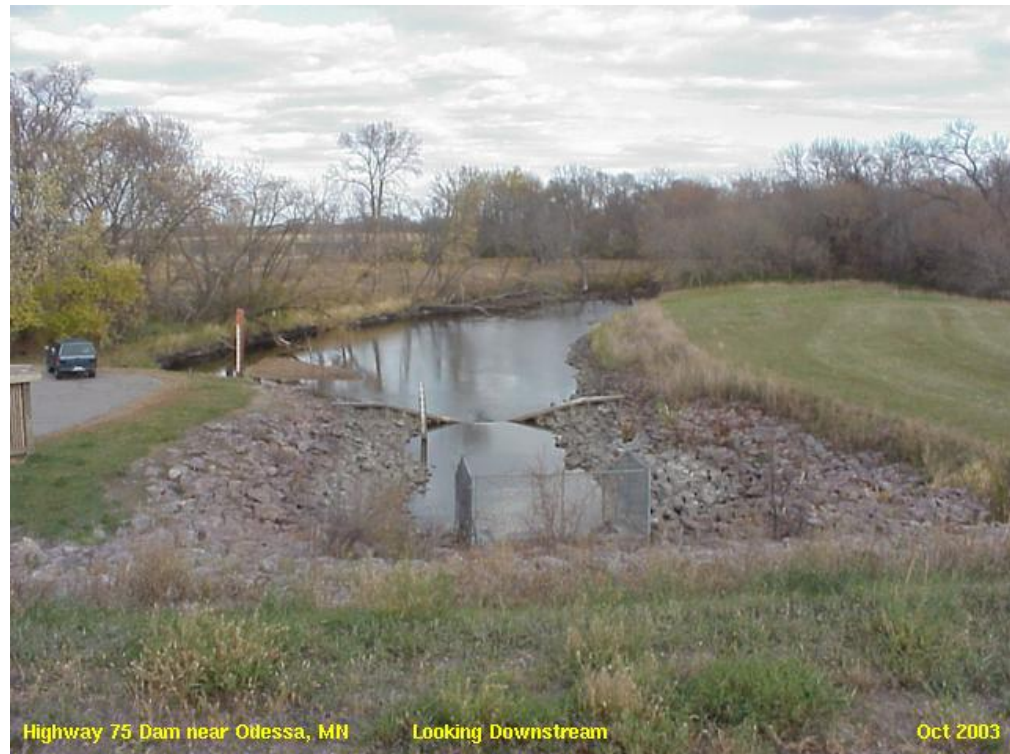
Figure 5-5. Highway 75 Dam Low Flow Outlet.
