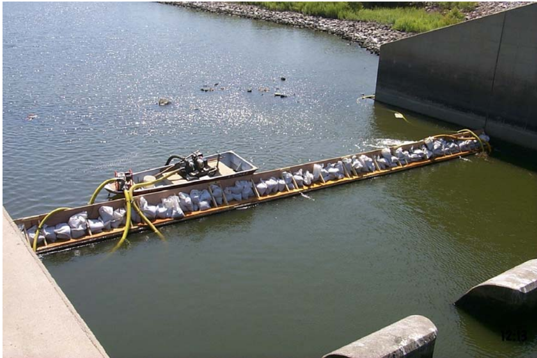
Figure 7-1. Periodic Inspection of the Bascule Leaf Gate Stilling Basin
