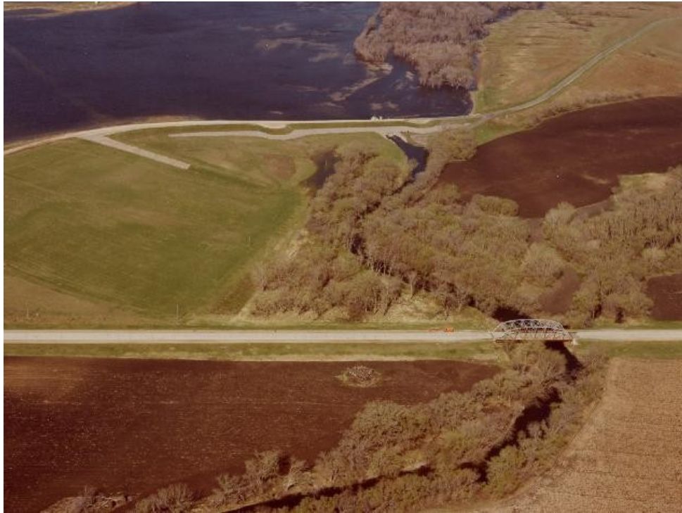
Figure 2-2. Emergency Spillway and Low Flow Outlet.
