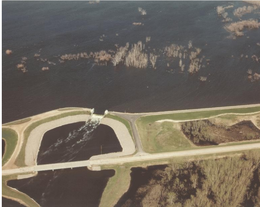
Figure 2-1. Highway 75 Dam Service Spillway
