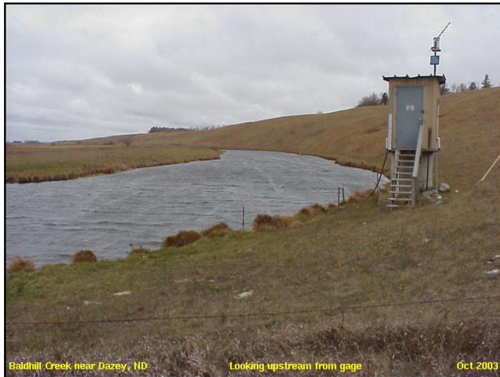
Figure 5-4. Dazey Gage on Baldhill Creek.
