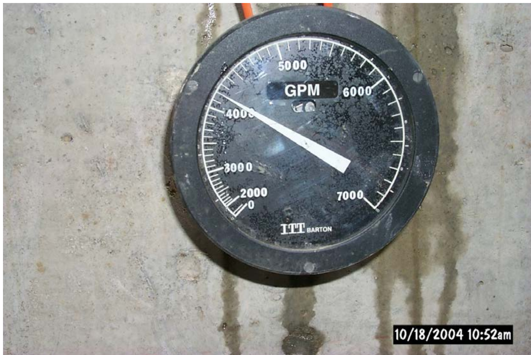
Figure 7-2. COE Water Meter to Monitor USFWS Demand
