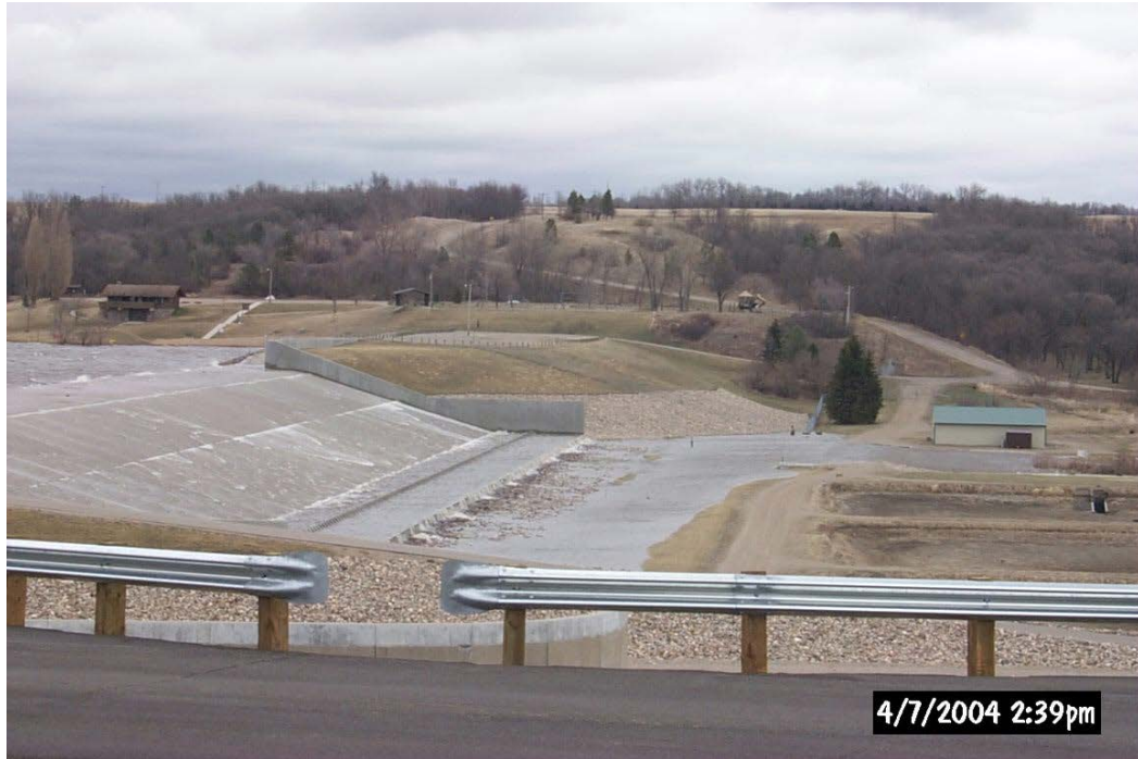
Figure 4-2. Baldhill Dam Flood Crest Spring 2004
