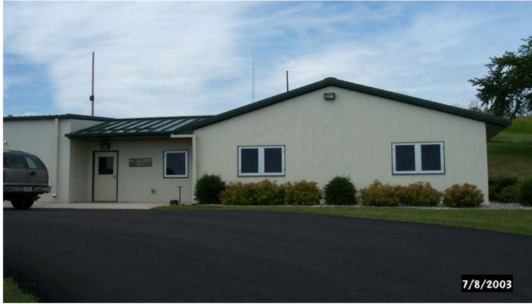
Figure 5-7. Baldhill Dam Project Office
