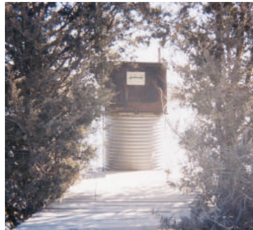
Figures 5-1 and 5-2. Lansing Stream Gage House
