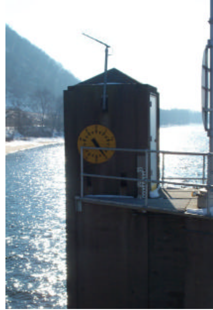
Figure 5-4. Tailwater Gage House
