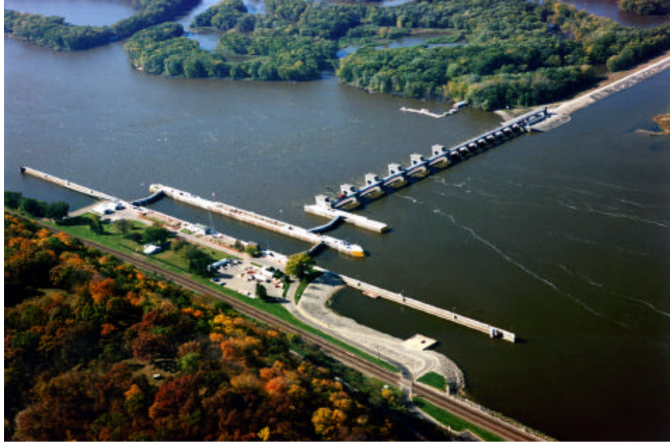
Figure 2-1. Lock and Dam No. 9
