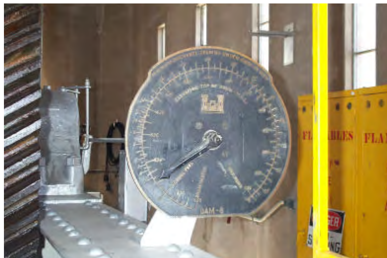
Figure 2-3. Alternate Roller Gate Position Indicator
