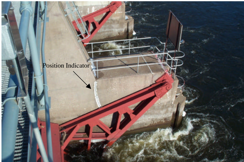
Figure 2-4. Tainter Gate Position Indicator
