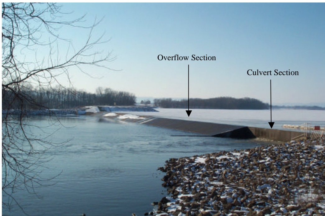
Figure 2-5. Onalaska Dam (looking west)
