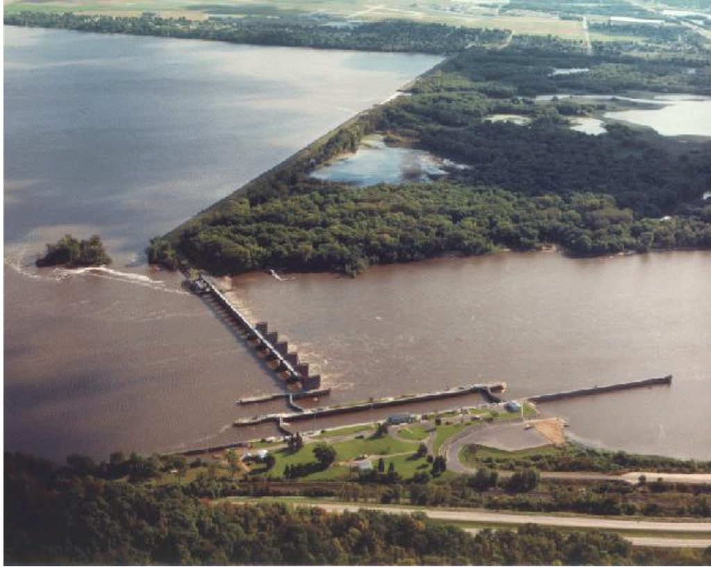
Figure 2-1. Lock and Dam No. 7 (looking east).
