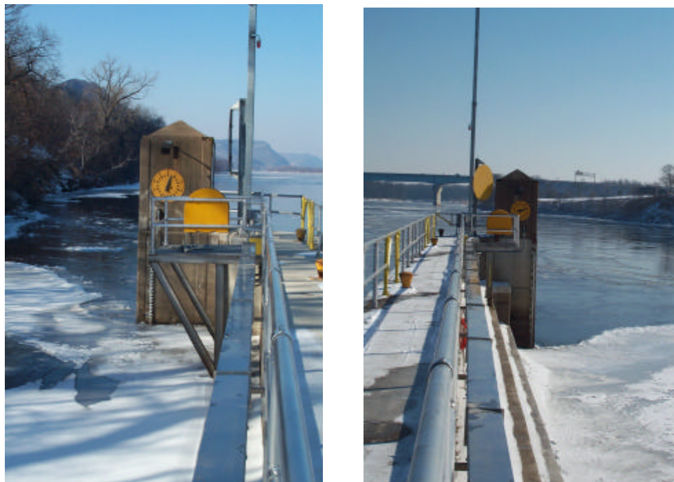
Figure 5-2. Pool (left) and Tailwater (right) gage houses
