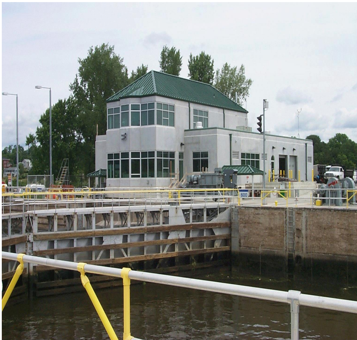
Lock and Dam No. 6 Control House Dedicated July 1999
