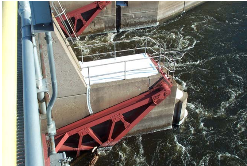
Figure 2-4. Tainter Gate Position Indicator
