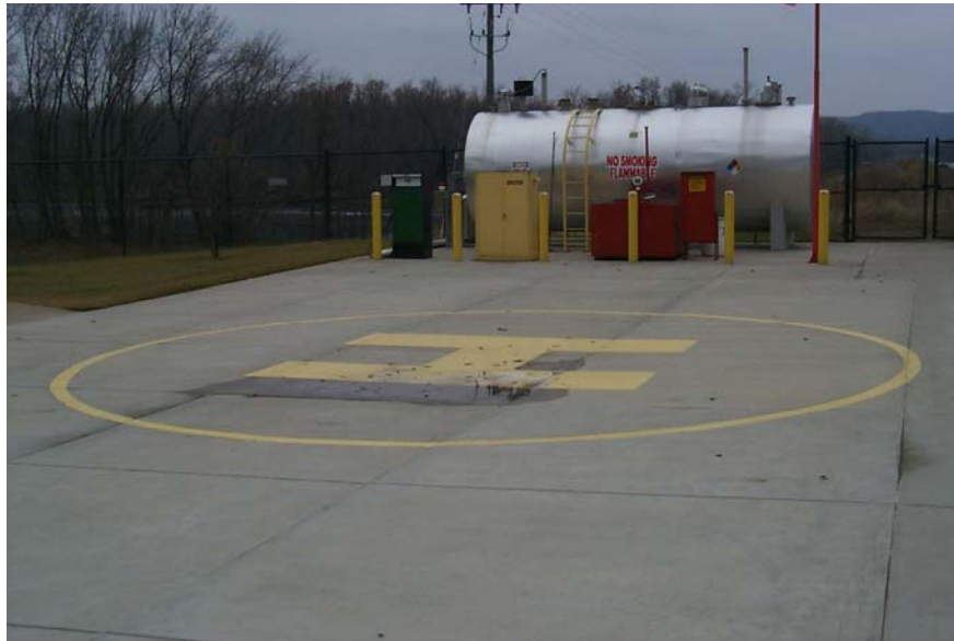
Figure 2-1. Helicopter Landing Pad behind the Central Control Station.
