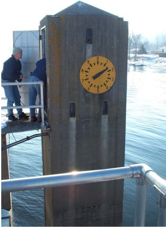
Figure 5-1. Control Point Gage House – Tailwater of Lock and Dam No. 5
