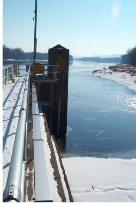
Figure 5-3. Tailwater Gage House
