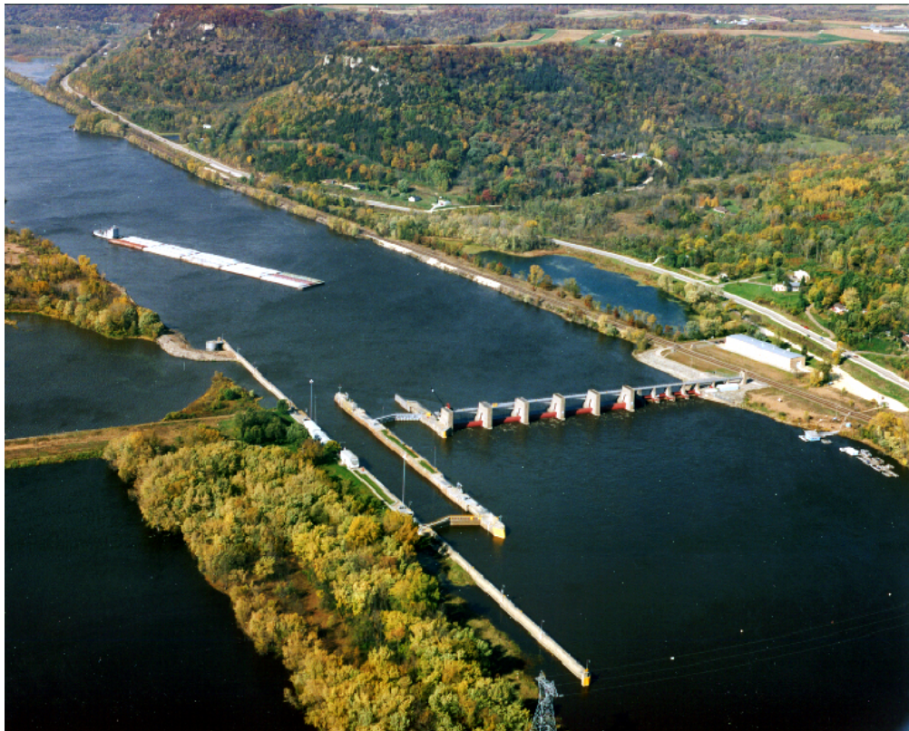
Figure 2-2. Lock and Dam No. 5A, October 1995 – Looking Upstream
