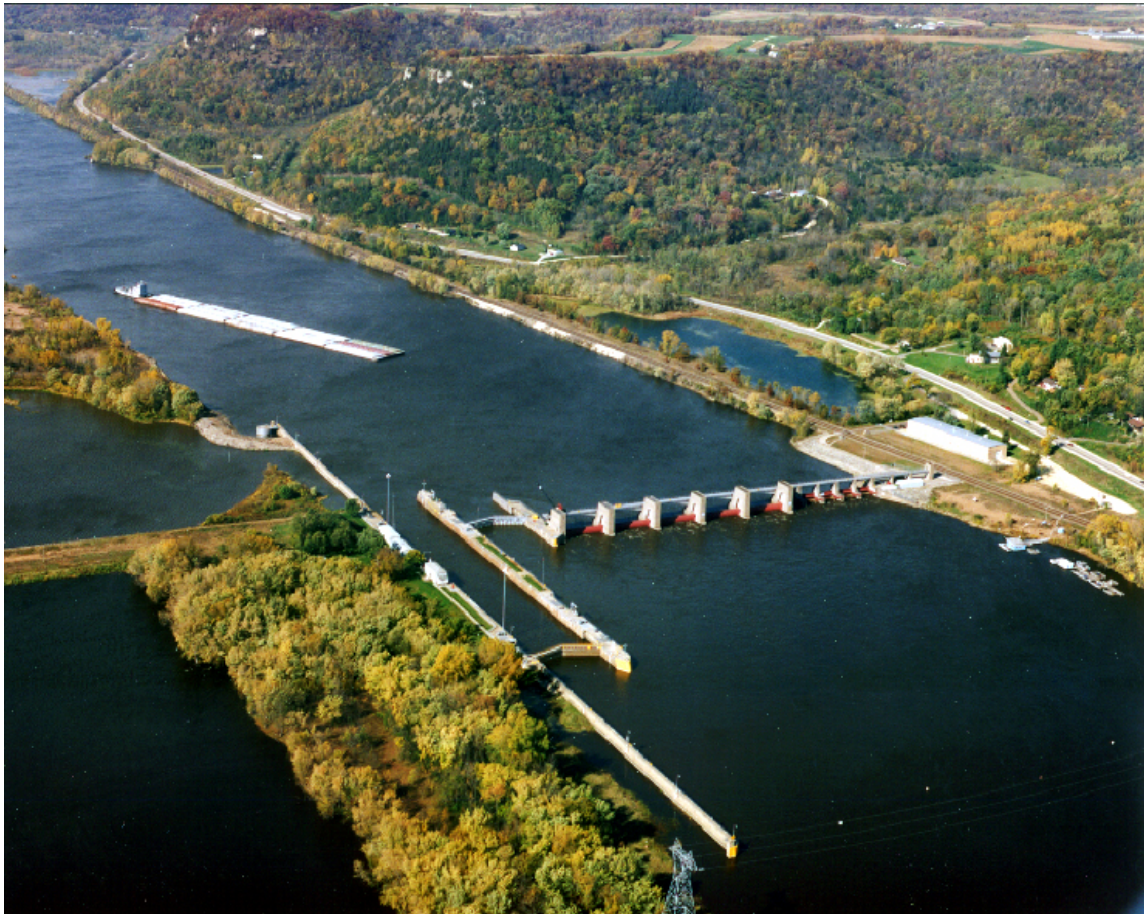
Aerial View Looking Upstream – October 1995
