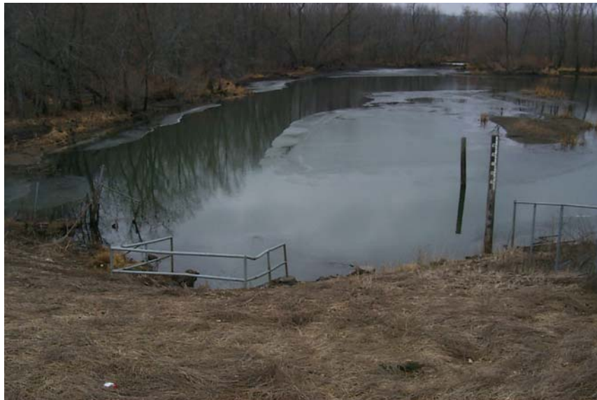
Figure 2-6. Prairie Island Control Structure Looking North at Crooked Slough
