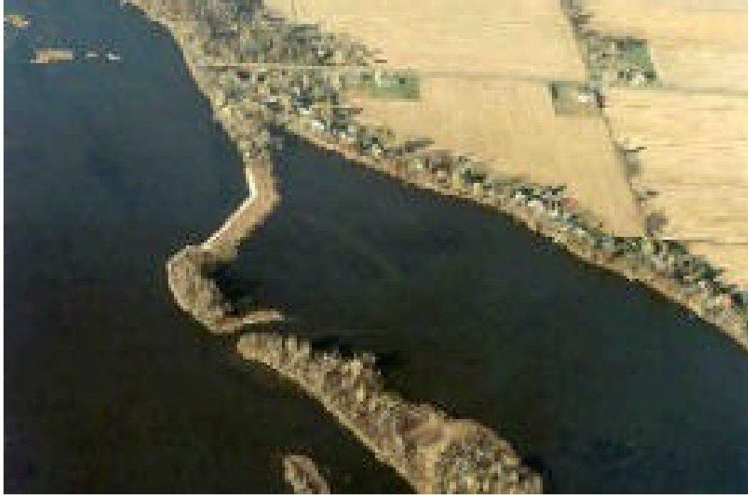
Figure 2-5. Breach Closure of Spring Lake Peninsula
