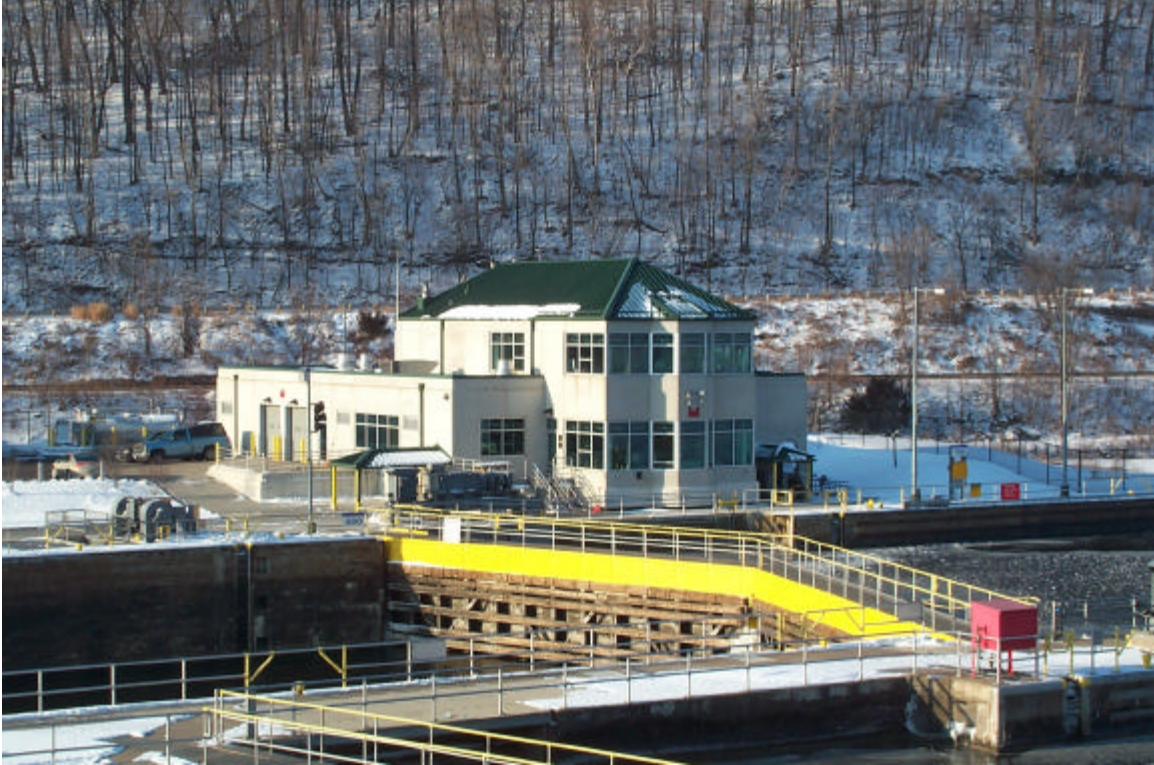
Lock and Dam No. 5 Control House Dedicated June 1998
