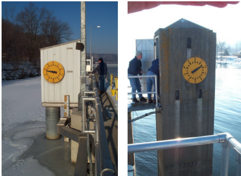
Figure 5-2. Pool (left) and Tailwater (right) Gage Houses
