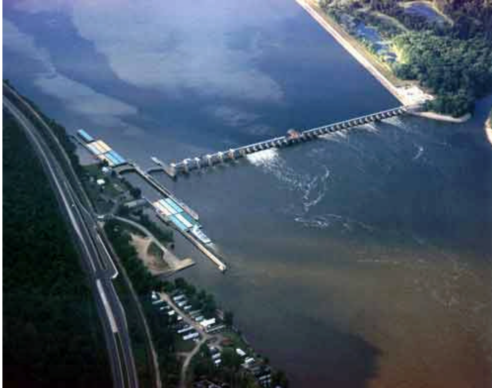
Figure 2-1. Lock and Dam No. 5 - Looking Upstream
