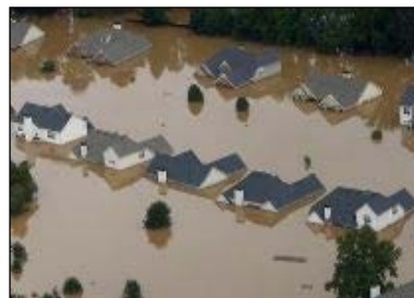
Sweetwater Creek, Austell, GA
