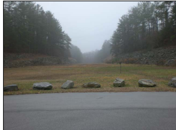
Figure 2-4. Spillway and Uncontrolled Chute
