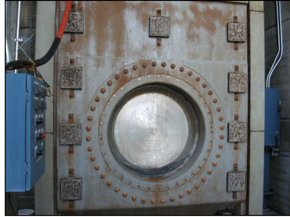
Figure 2-6. Broome-type Sluice Gate
