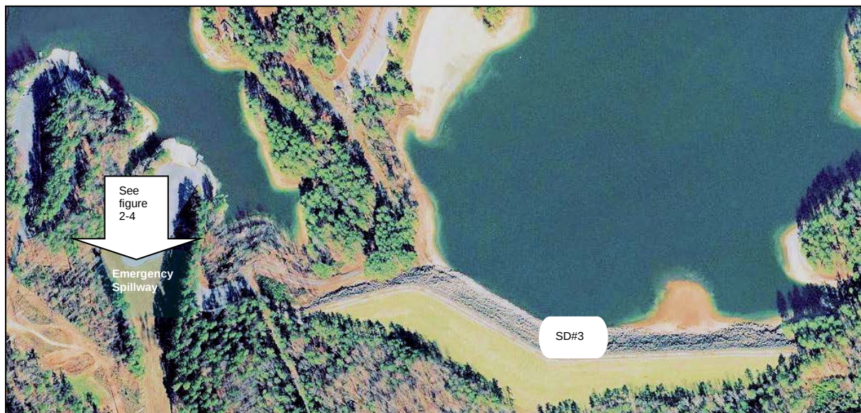
Figure 2-3. Saddle Dike No. 3 and Emergency Spillway
