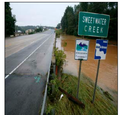
Sweetwater Creek flooding
