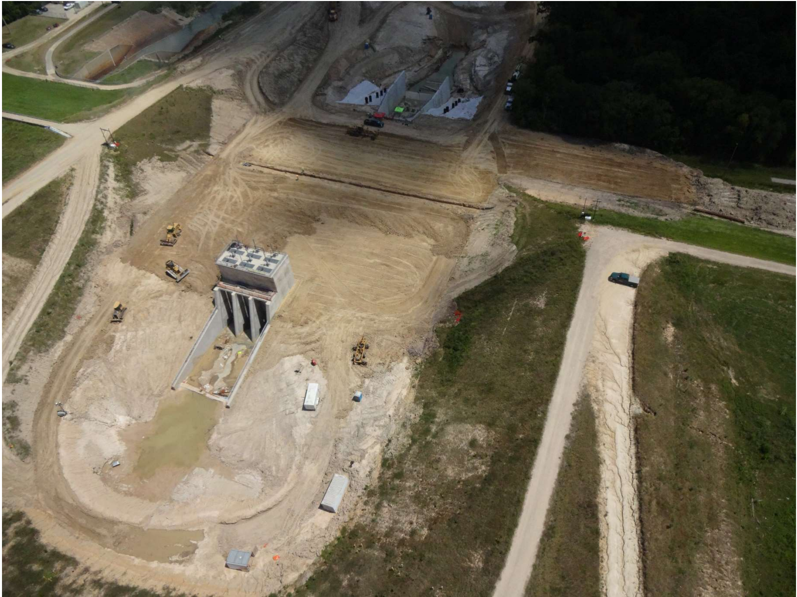
ADDICKS RESERVOIR – OUTLET WORKS (AUGUST 2019)
