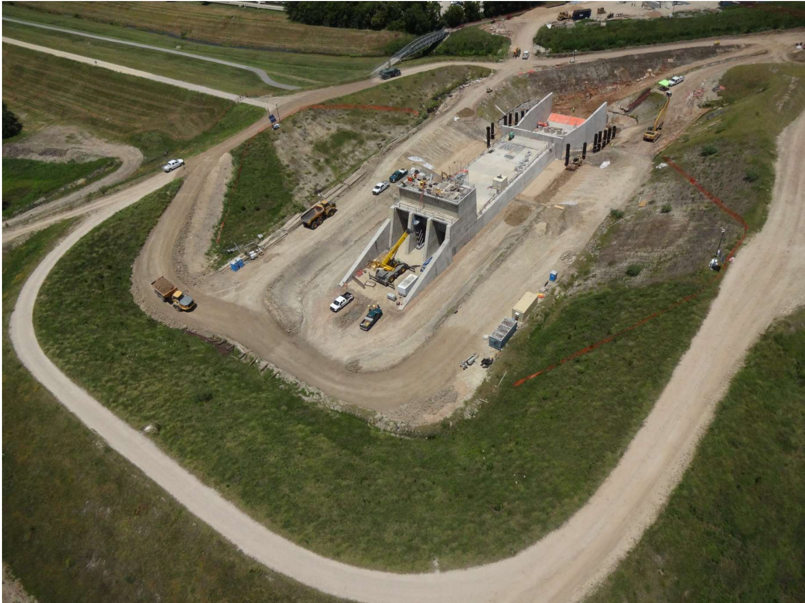
BARKER RESERVOIR – OUTLET WORKS (AUGUST 2019)
